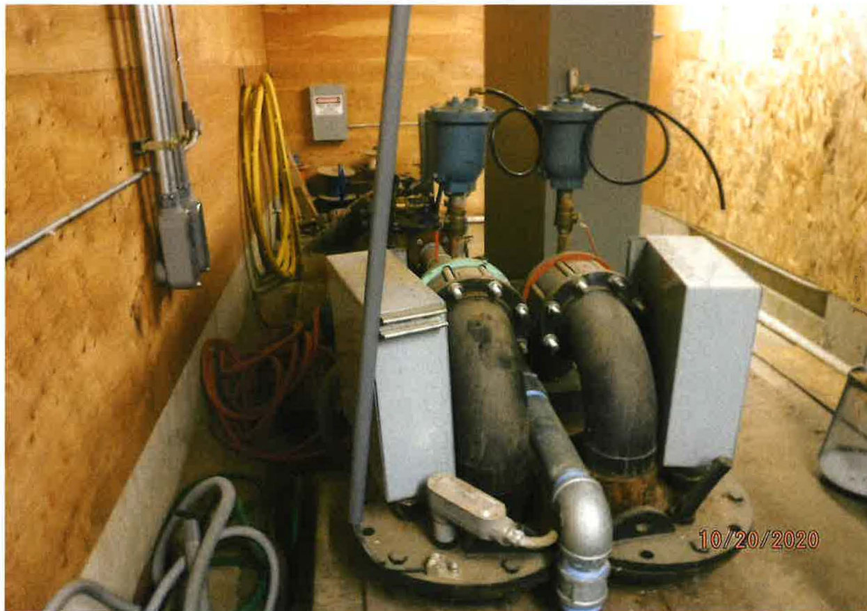
POD – PRE 1960 WELL – NO IDENTIFICATION, LOCATED IN THE NESESW 50N04W SECTION 3
