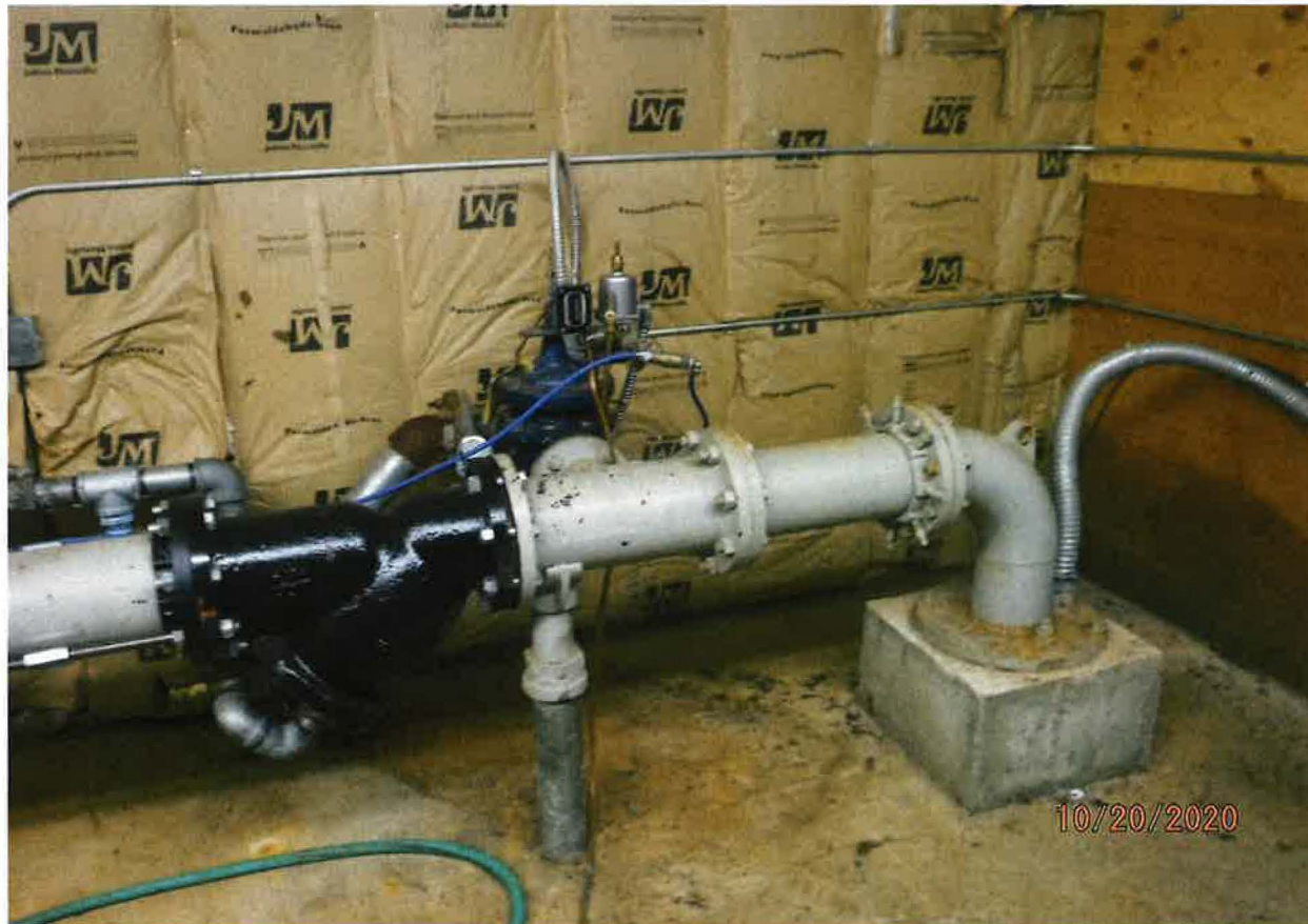
POD – WELL 95-95-C-0008, 75 HP PUMP INSTALLED
