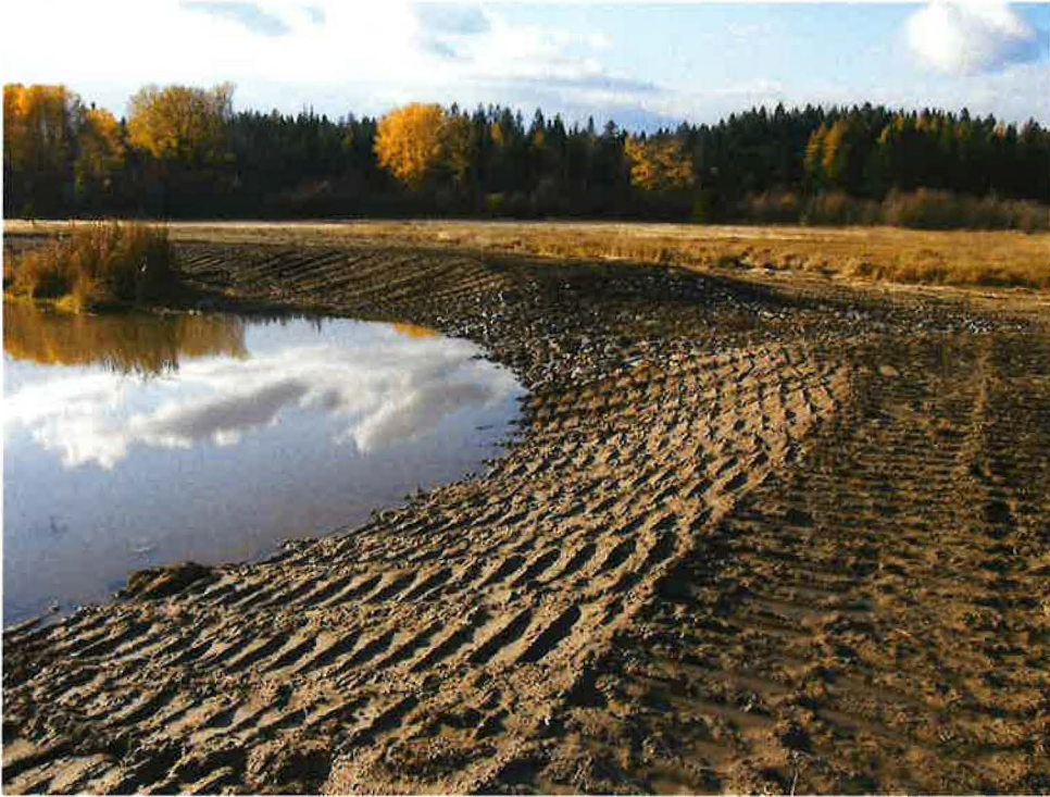
Photo 9. Dike after construction, facing the spillway (November 2015).
