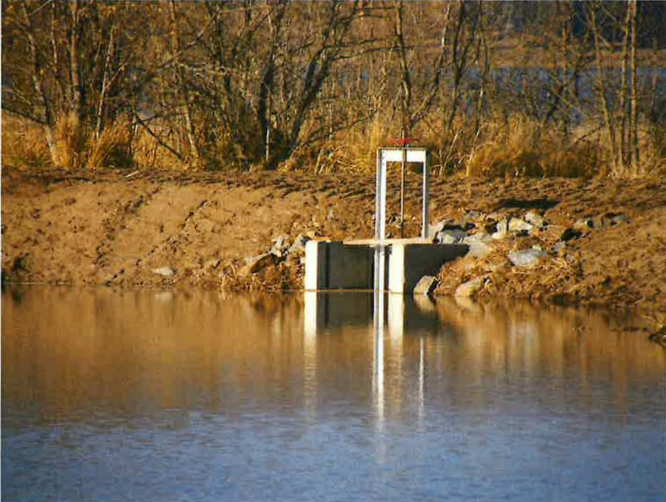
Photo 8. Dike with water control structure after construction (November 2015).
