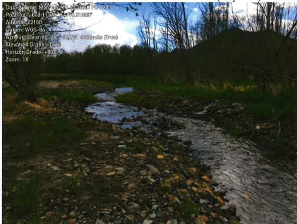
Photo 14. Rock drop chute constructed between wetlands (May 2017).
