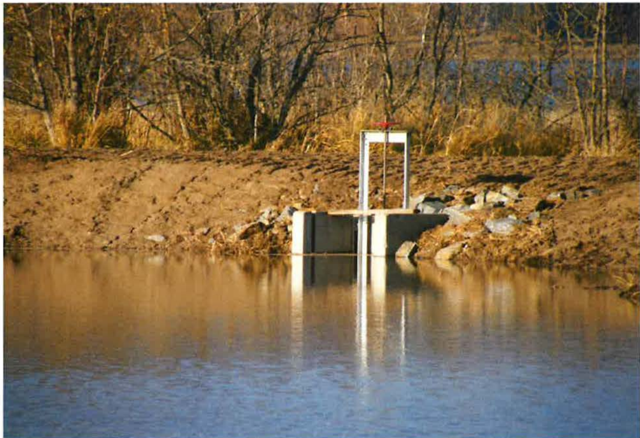
POD – CONCRETE HEADGATE ALONG POND # 1 (PHOTO PROVIDED BY IDAHO FISH AND GAME)
