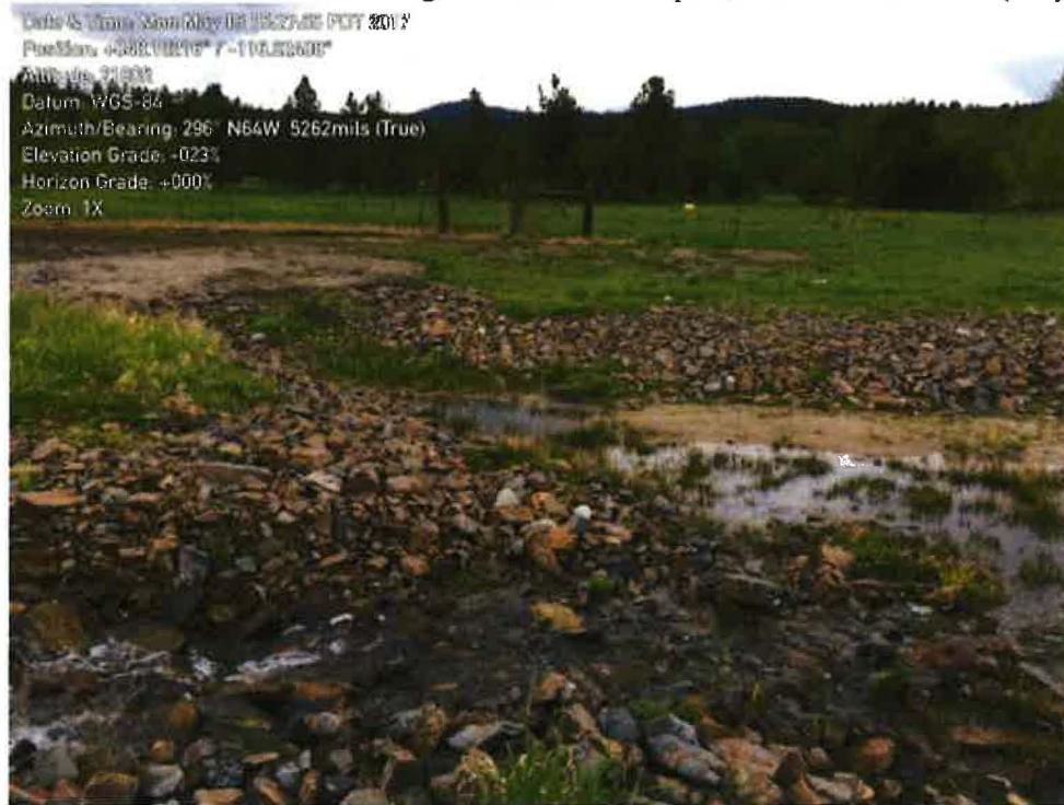
Photo 13. Excavation 6 showing rock added for repair, after erosion event (May 2017).
