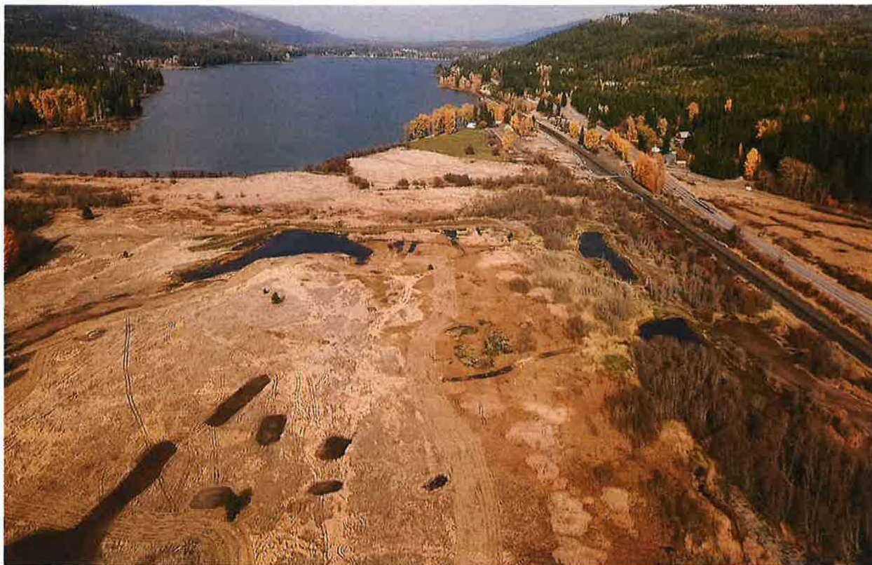
AERIAL OVERVIEW PONDS 1-3 WILDLIFE STORAGE, RECREATION STORAGE, AND FIRE PROTECTION STORAGE POU
