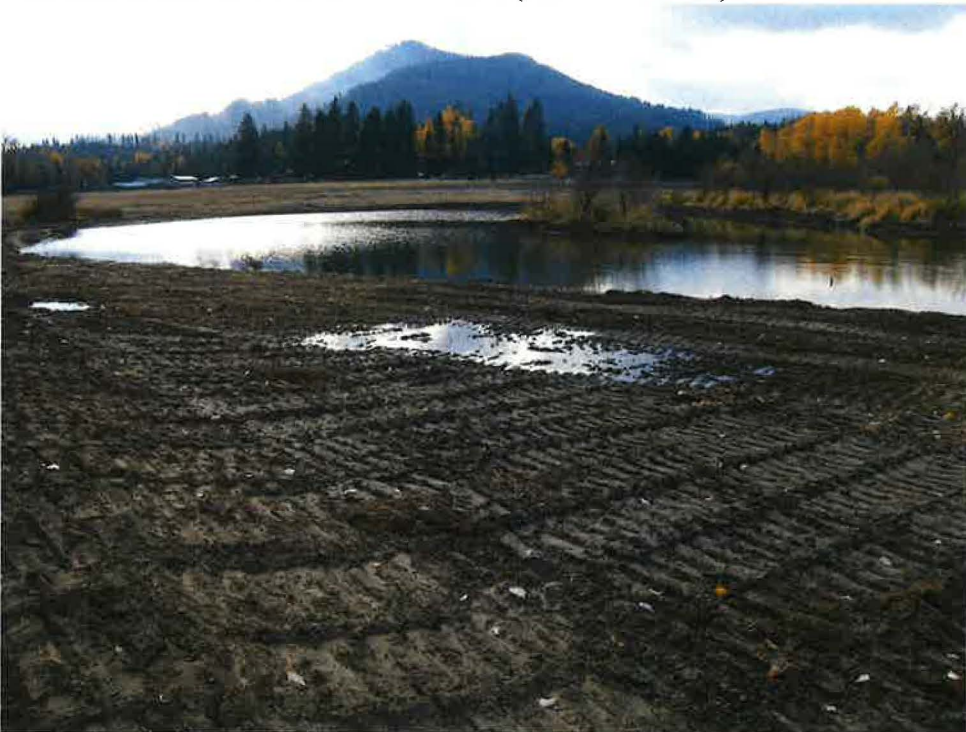
Photo 10. Excavation 5 after construction (November 2016).
