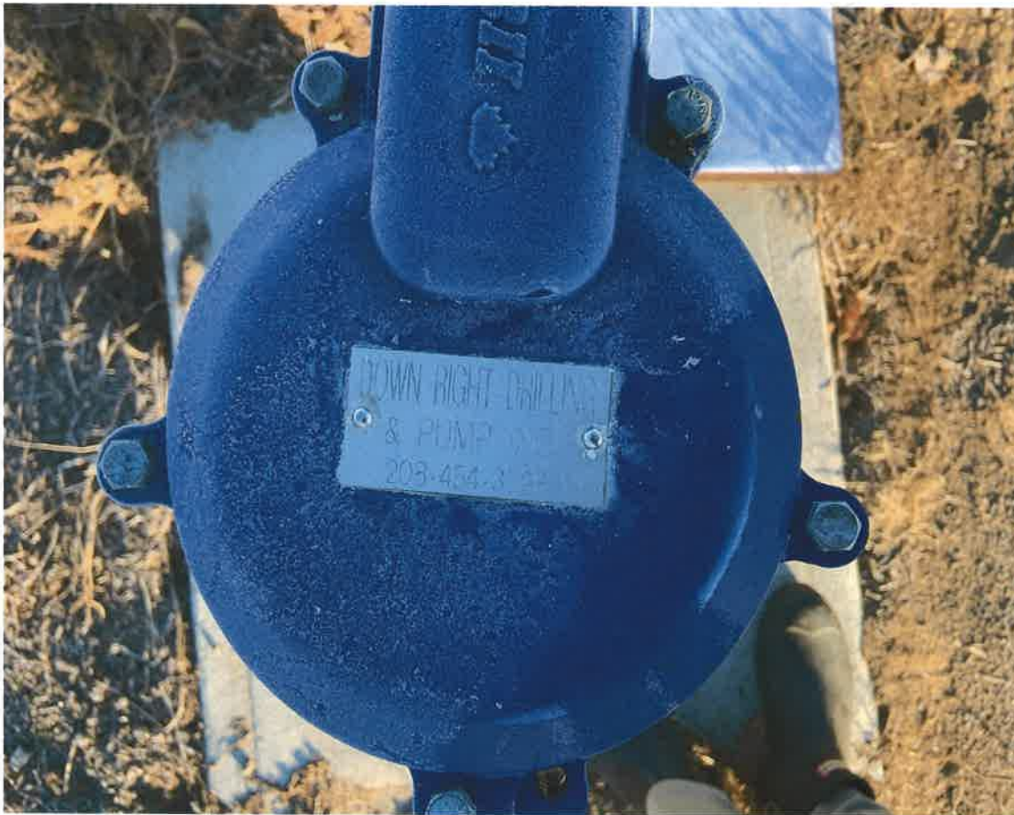
Fig. 3 – Well drilling and pump instillation was done by Down Right Drilling & Pump.
