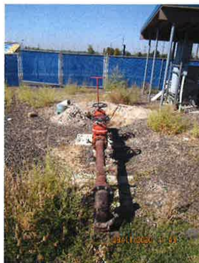
Small section of the well diversion pipe that exists above ground.
