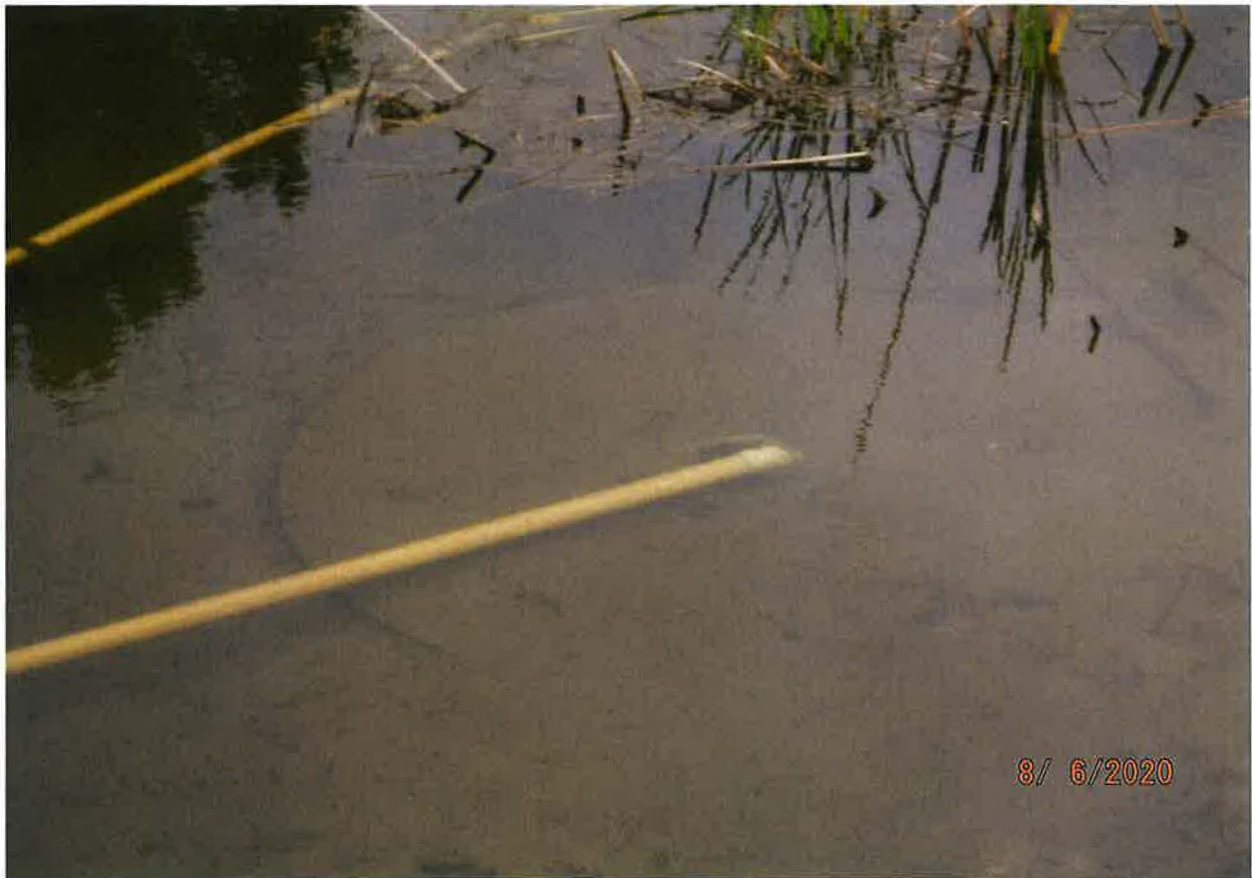
IRRIGATION FROM STORAGE SYSTEM AT POND POU
