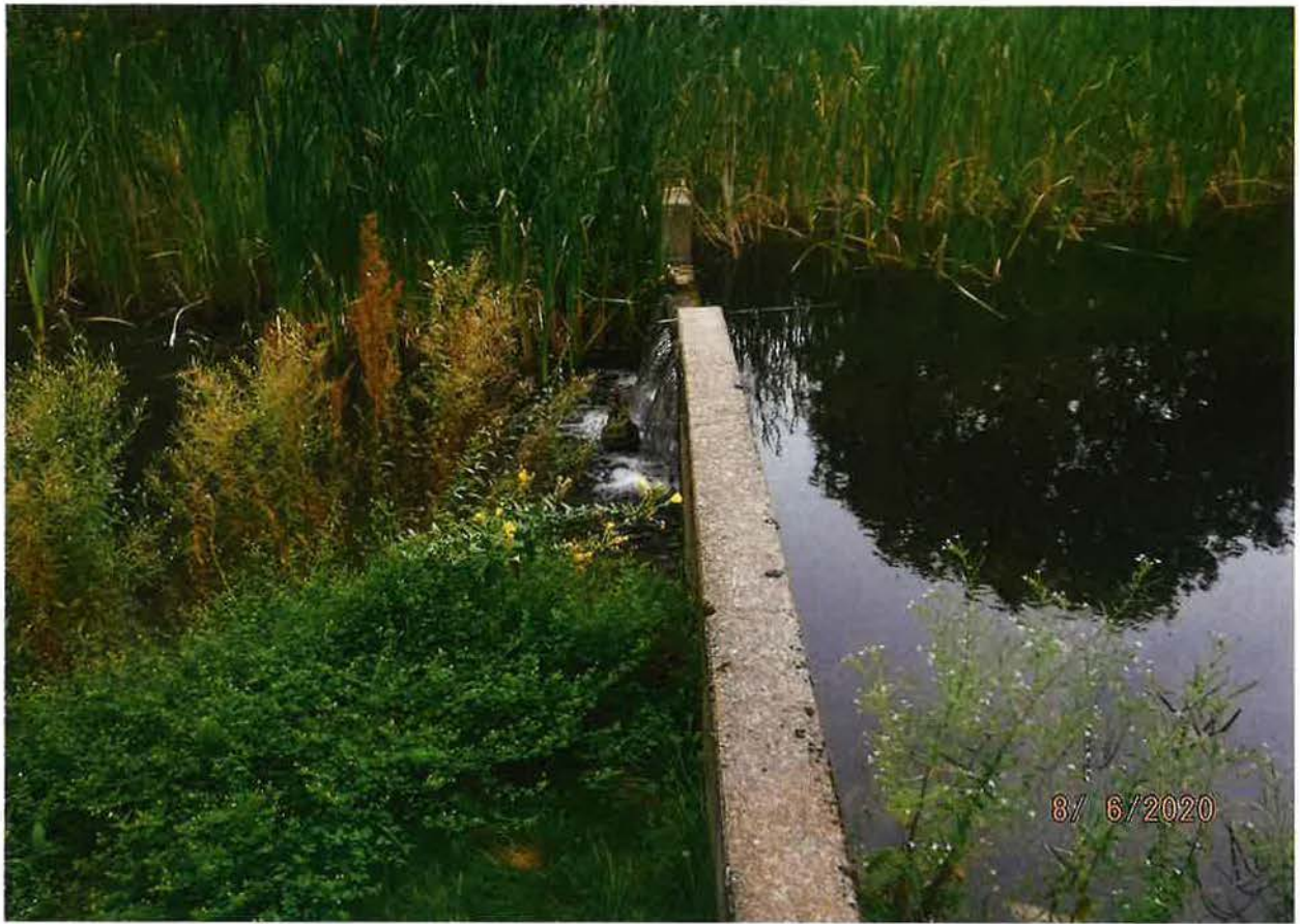
WATER LEVEL CONTROL POINT IN POND
