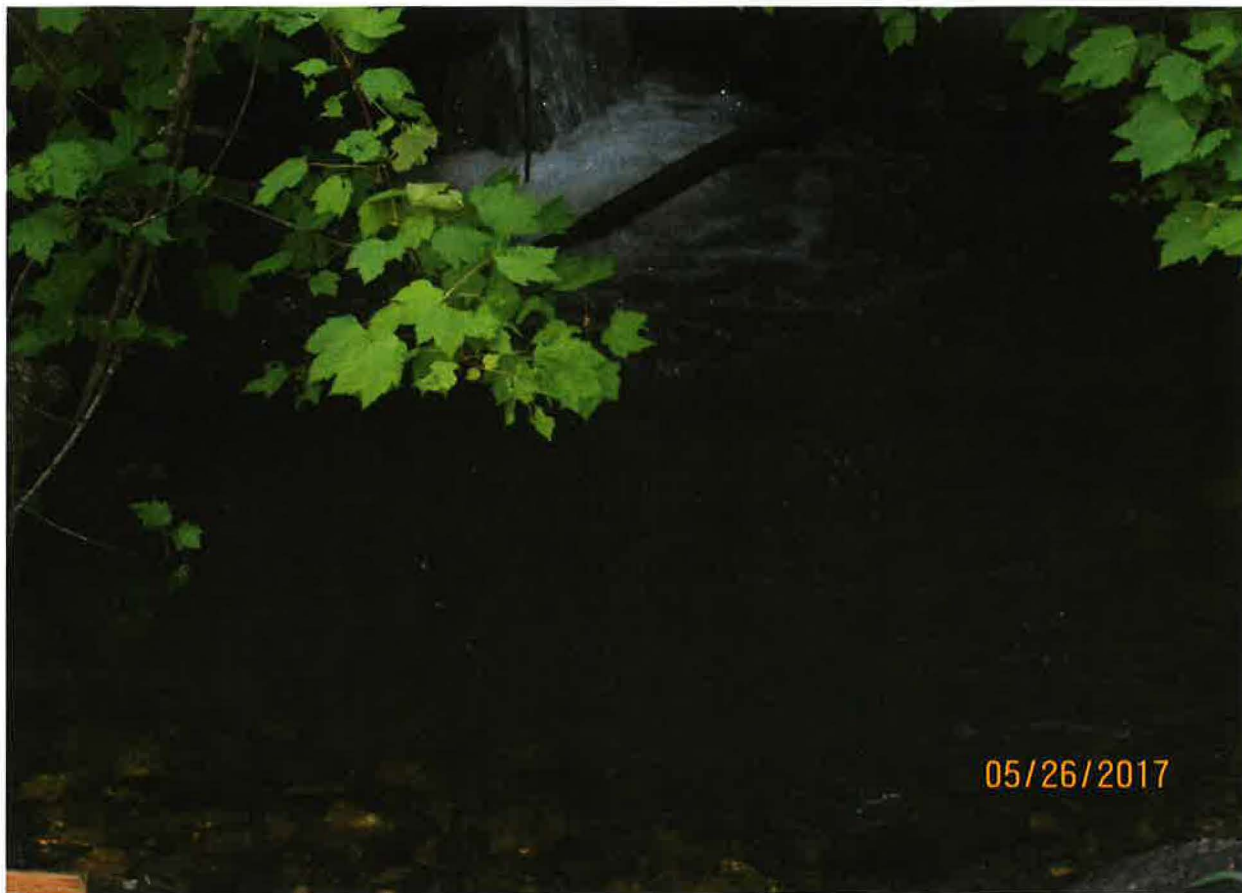
POD – INTAKE PIPE IN UNNAMED STREAM, SHOWN AT HIGHER WATER LEVEL SPRING
