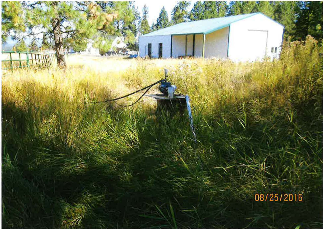
1 HP STA-RITE PUMP FROM STORAGE TANK TO IRRIGATION AND STOCKWATER USE(S)
