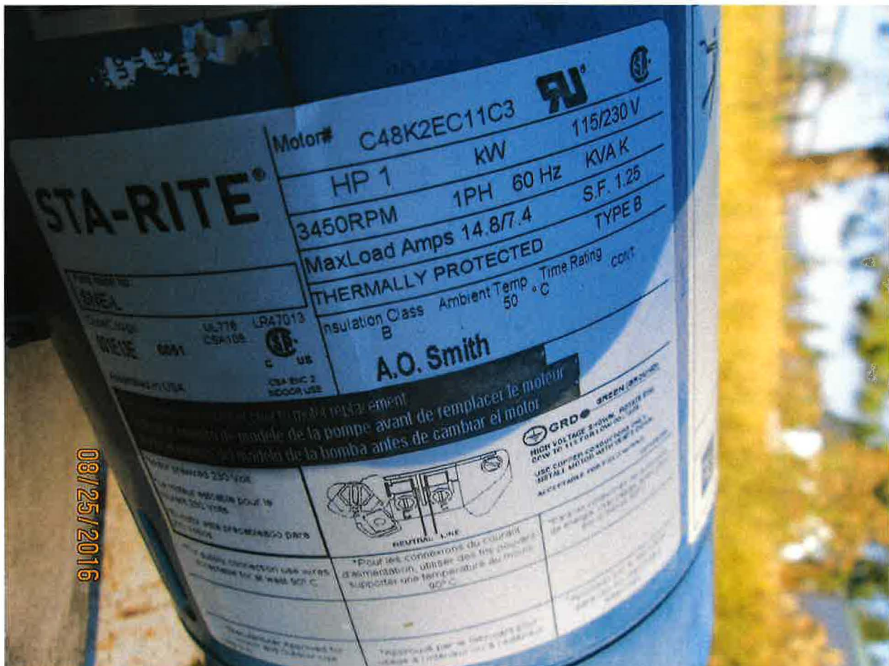
1 HP STA-RITE PUMP FROM STORAGE TANK TO IRRIGATION AND STOCKWATER USE(S)
