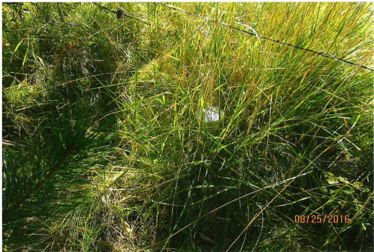
SPRING POD – BURIED SPRING BOX WITH VENT PIPE
