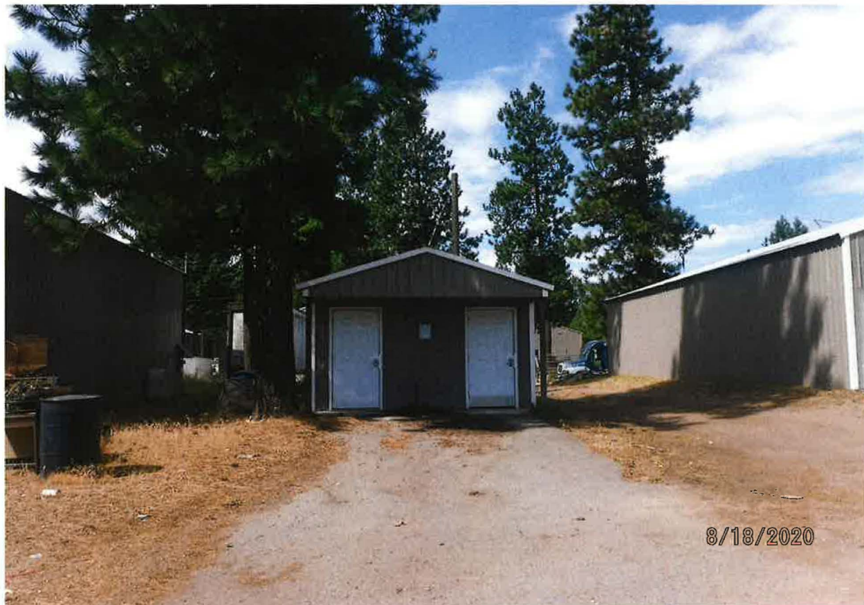
DOMESTIC POU – CENTRAL POINT RESTROOMS AND OFFICE BLDG RESTROOMS
