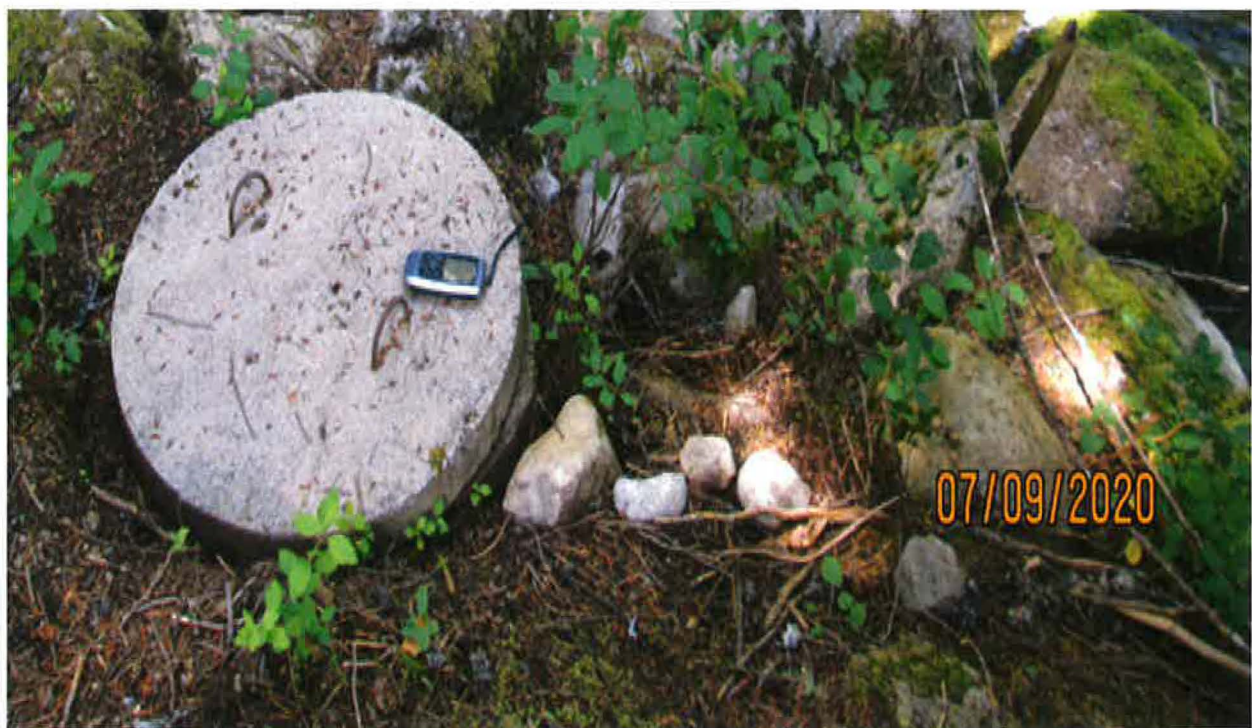
POD – CONCRETE CISTERN THAT INTERCEPTS GROUNDWATER AS IT FLOWS TOWARD CARR CREEK
