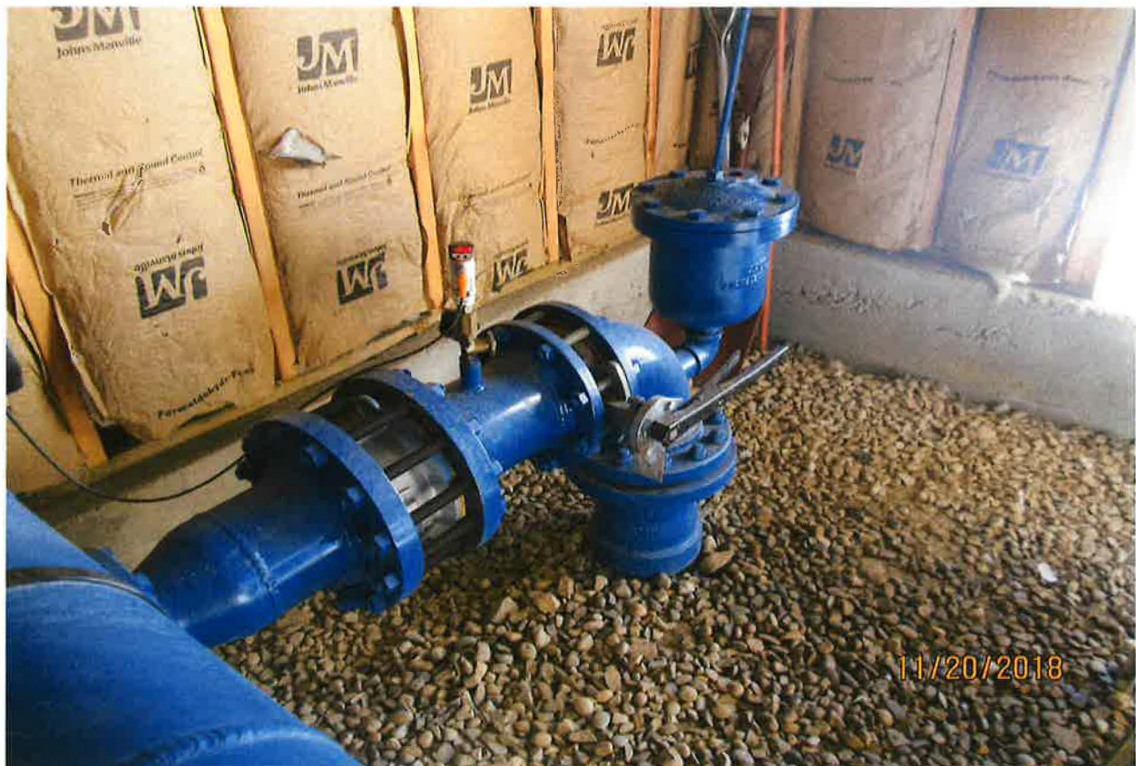
WATER CONVEYANCE SYSTEM
