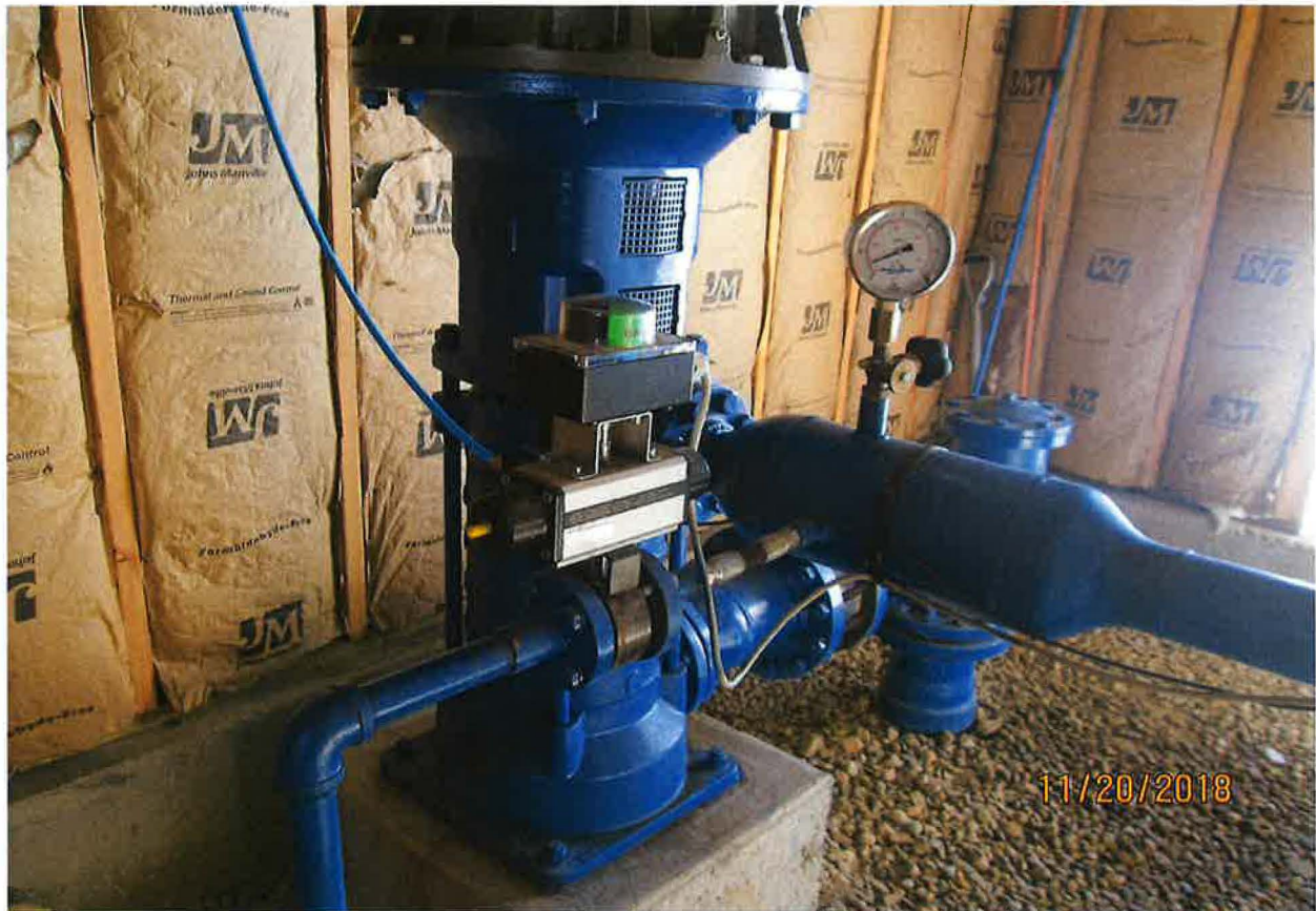
200 HP BALDOR MOTOR – BOOSTER PUMP
