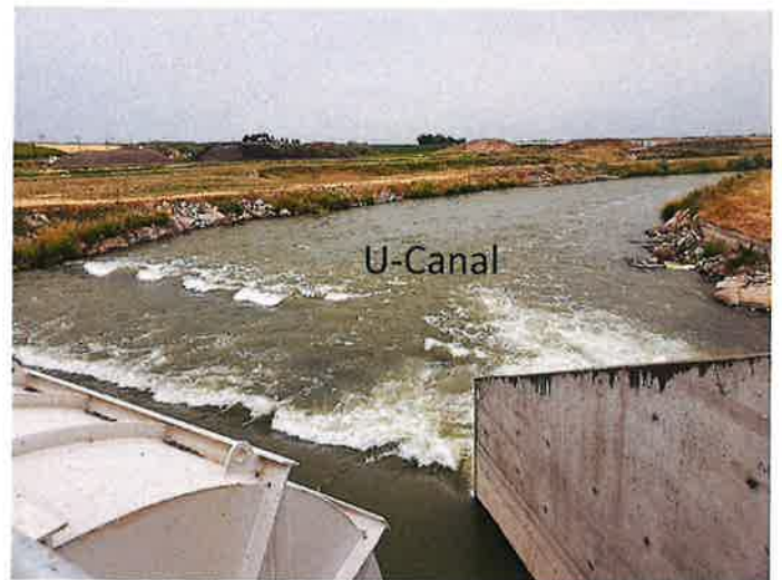
U-Canal, downstream view, Northwest direction
