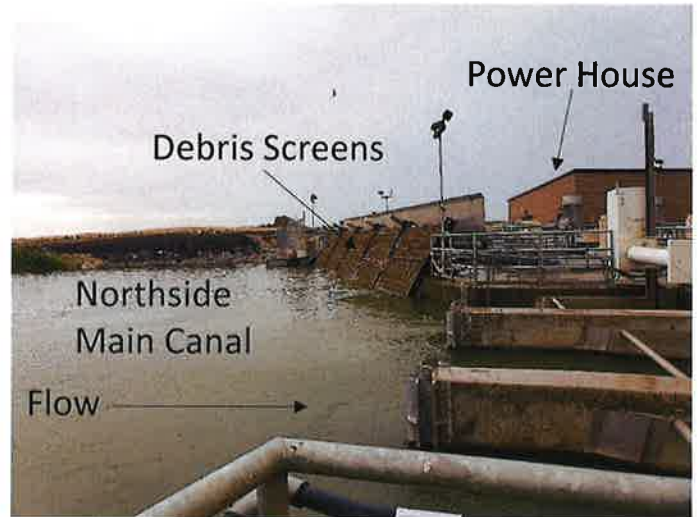
Northside Main Canal, upstream side, with debris screens and view of power house
