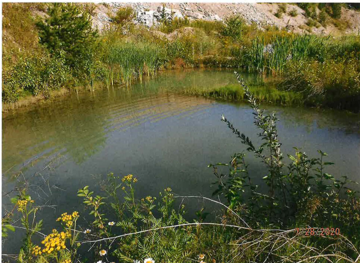
SMALL SETTLING POND FOR SILT FALL OUT BEFORE ENTERING STORAGE POU
