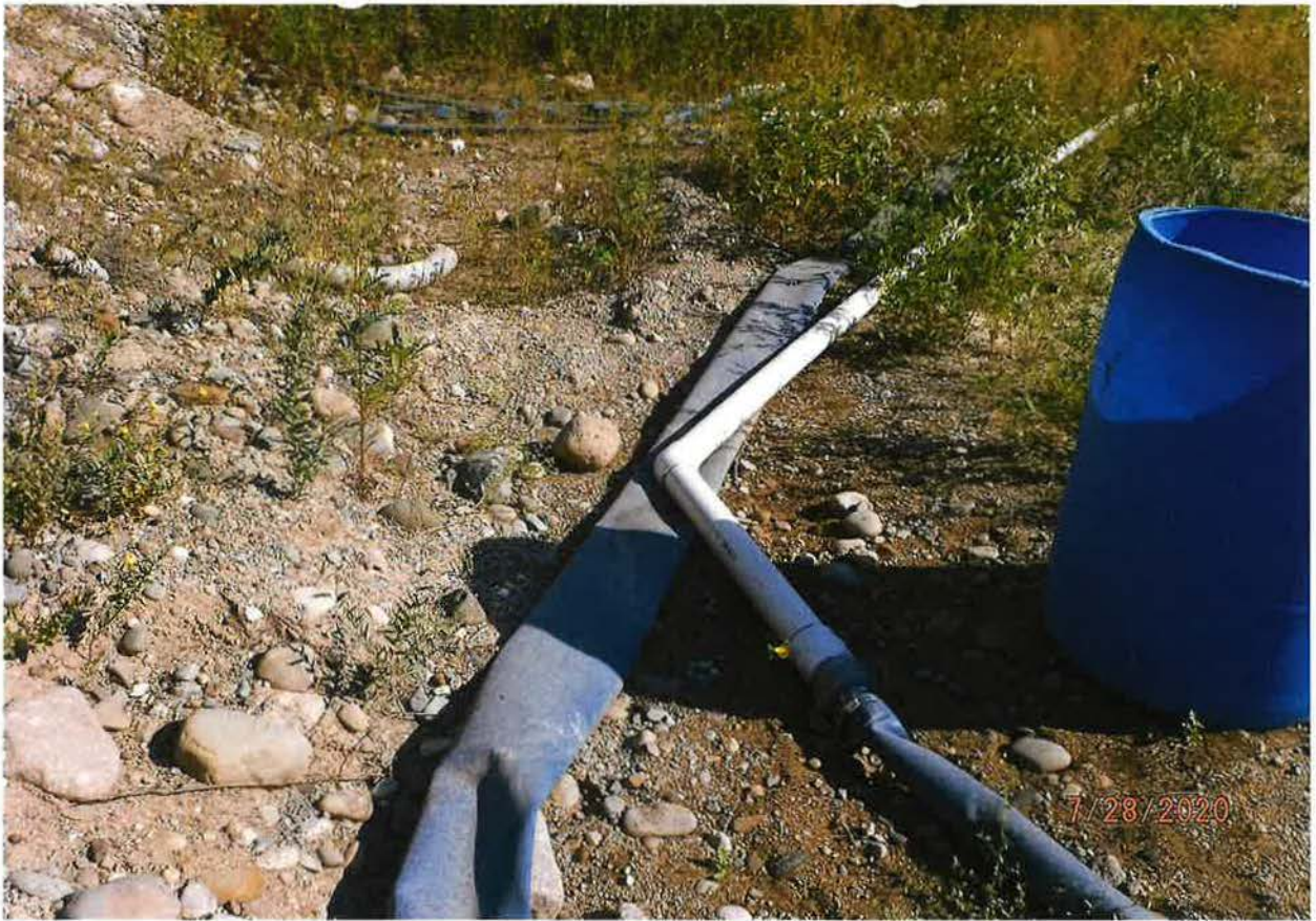
WATER CONVEYANCE FROM POD TO SETTLING POND
