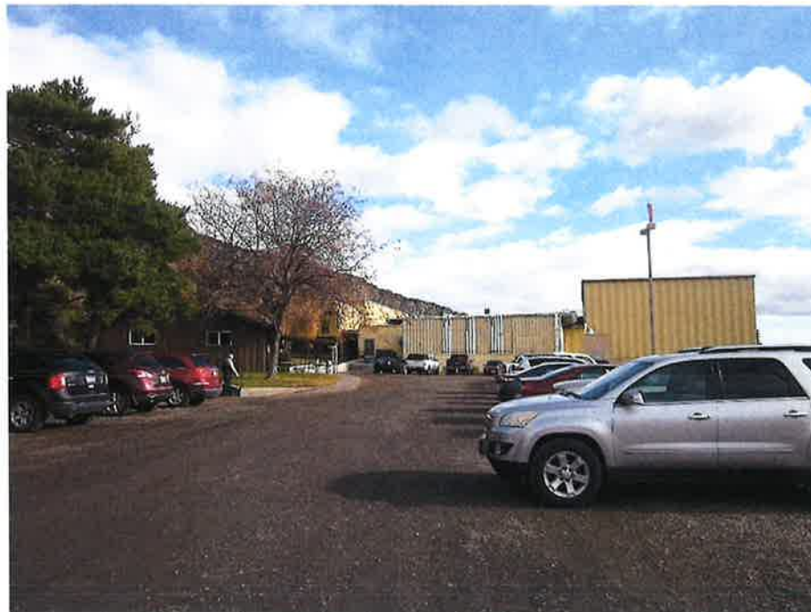
Figure 6: Looking east at processing plant and break room (on the left)
