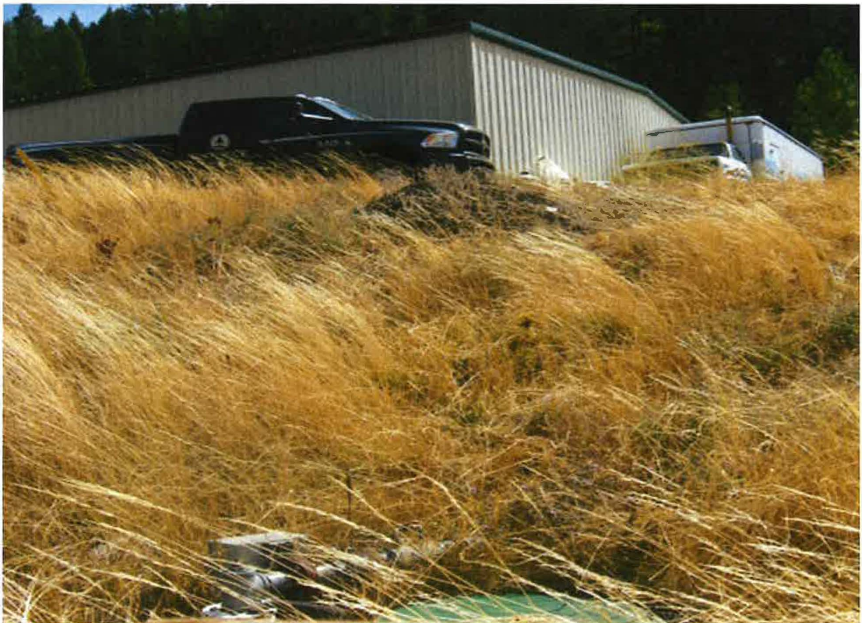
FIRST STAGE PUMP HOUSE FOR WATER SYSTEM
