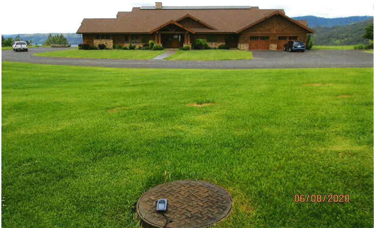
DOMESTIC POU – MAIN RESIDENCE
