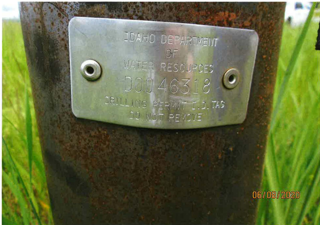
POD – WELL D0046318
