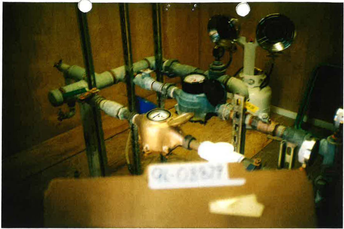
Inside Pump house
