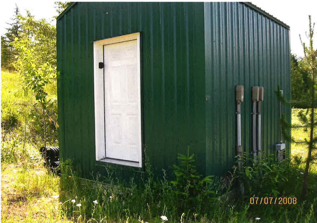
WATER SYSTEM PUMP HOUSE
