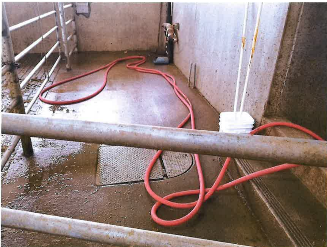
Looking at one of four deck flush holes. Applicant says deck flush is not used and water from a 10,000 gallon holding tank is used.
