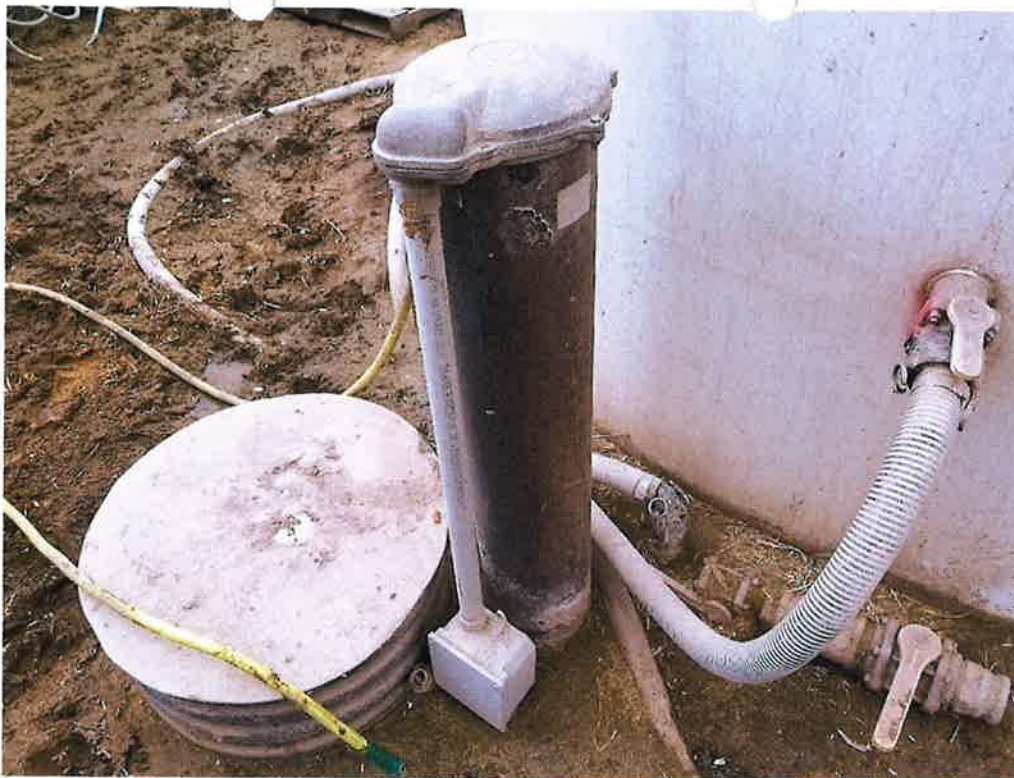
Looking at well (No “D” Tag)
