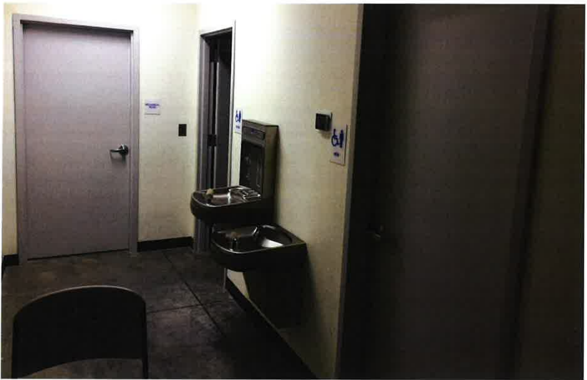
Administration building restrooms and drinking fountains
