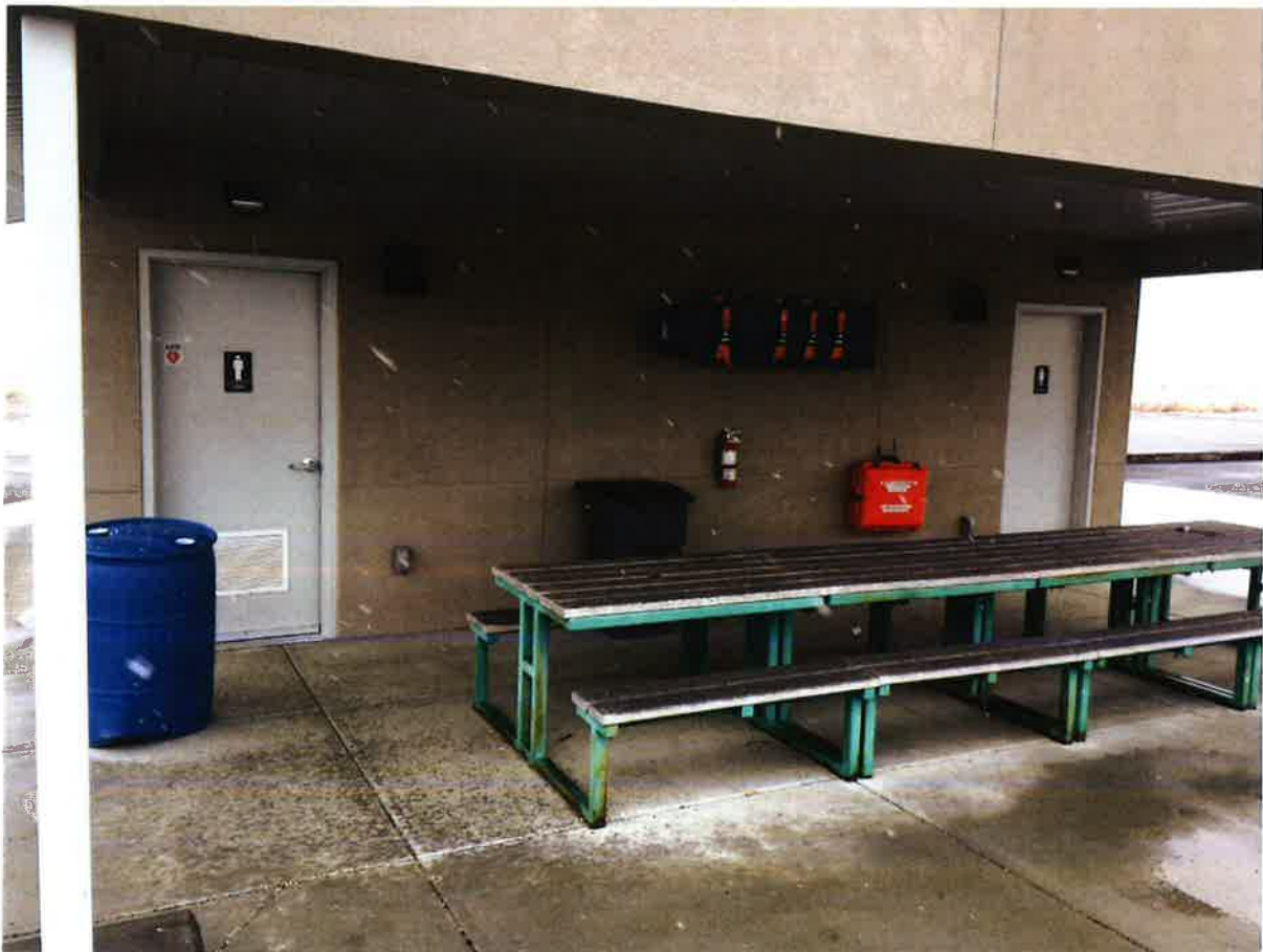
Satellite restroom building.
