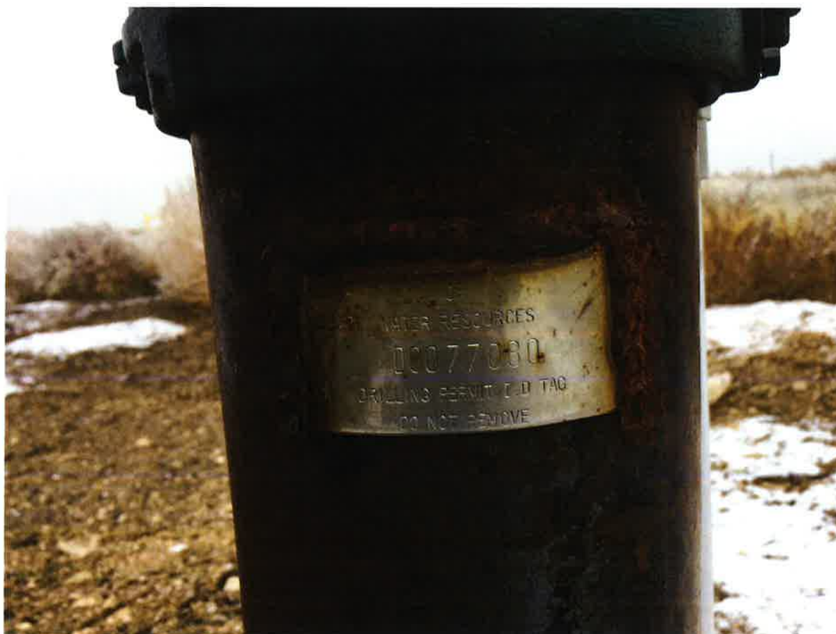
Well casing with tag No. D0077080.
