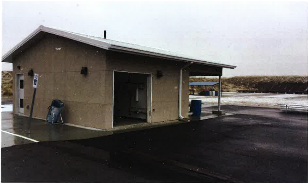
Satellite restroom building. Hose bib adjacent to roll up door.
