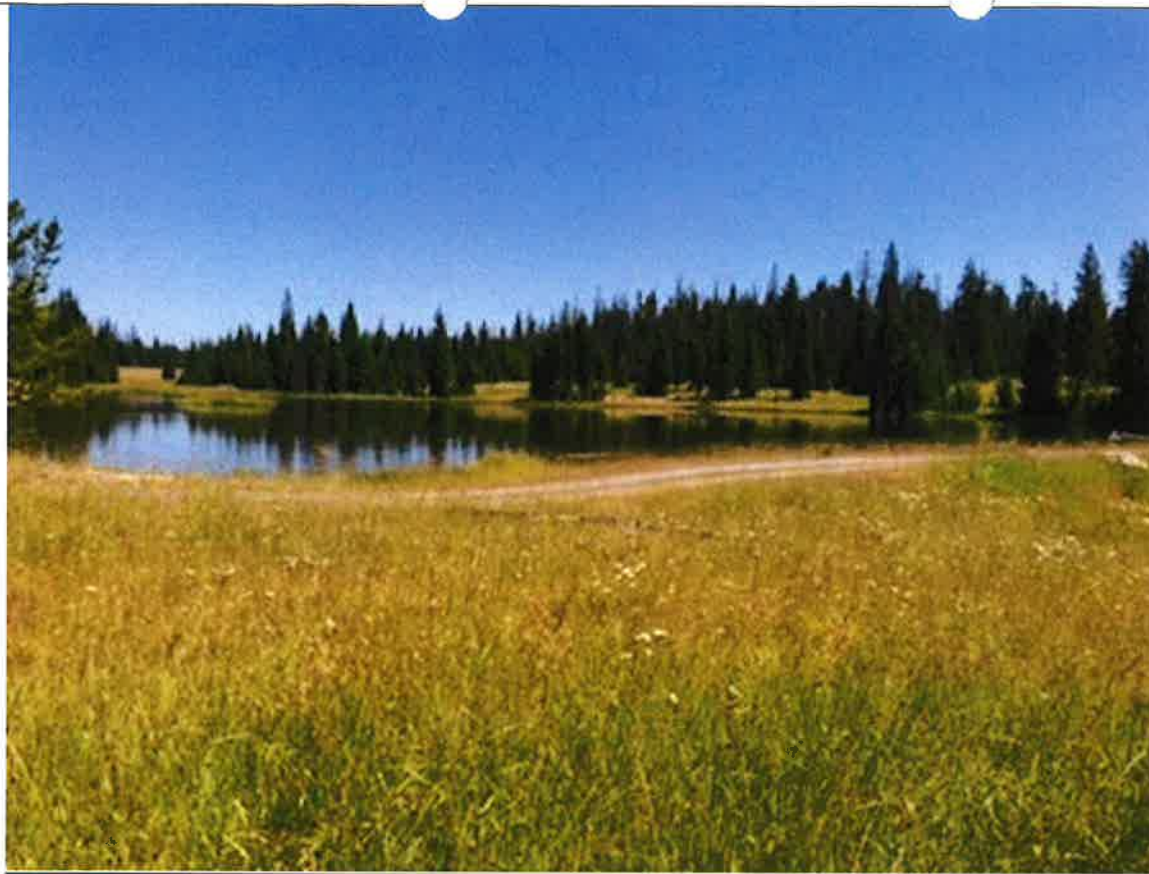
Figure 3. Looking NE across dam at pond.
