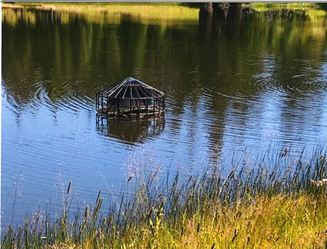
Figure 2. Overflow drain.
