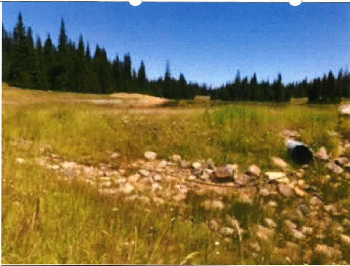
Figure 5. Overflow outlet culvert on downstream side of dam.
