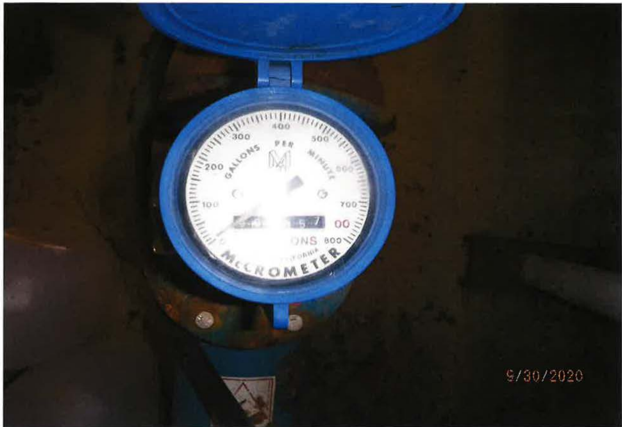
WATER SYSTEM FLOW METERS
