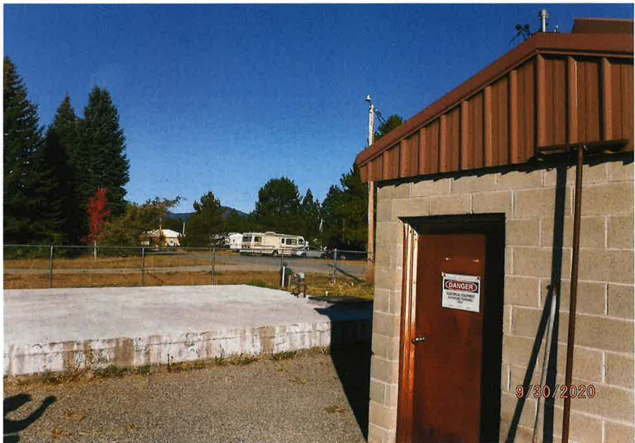
AT POD – PUMP HOUSE, STORAGE TANK, AND WELL
