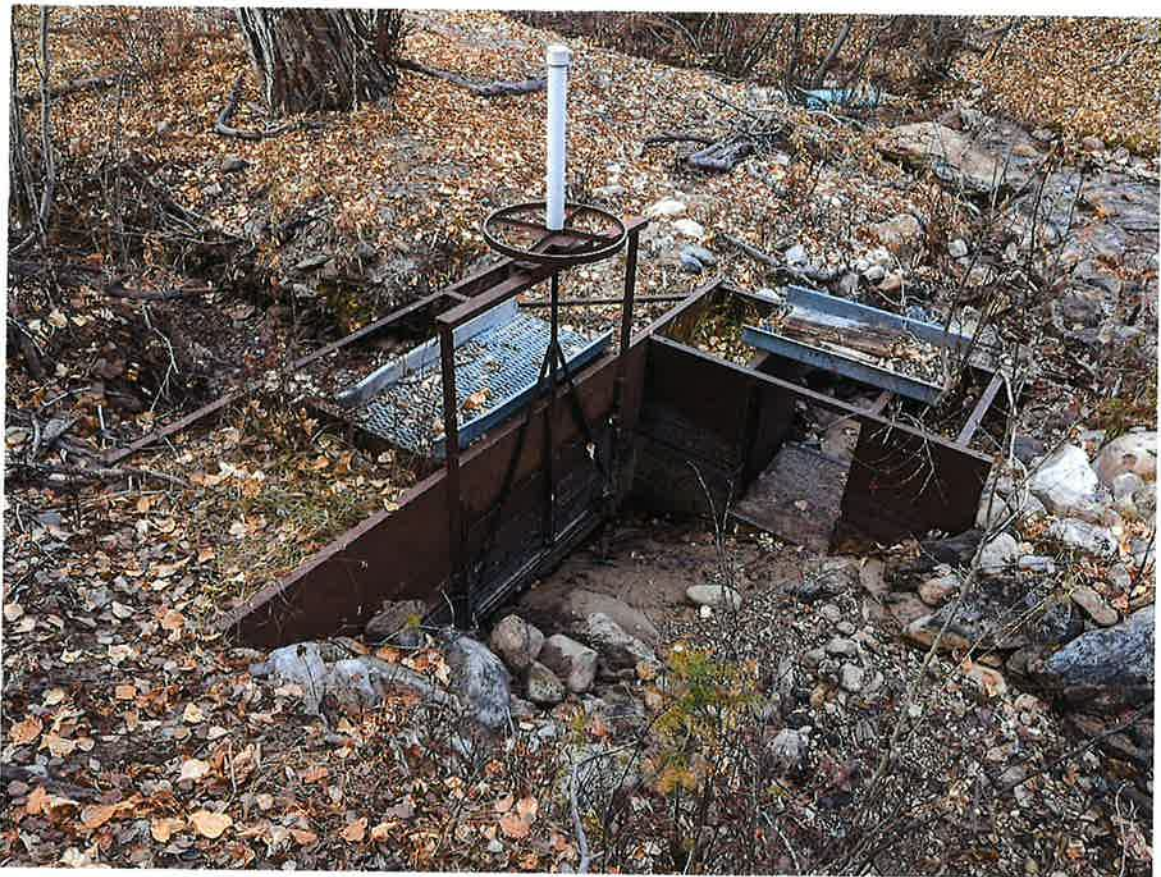
Photo 1: Diversion on Freeman Creek
