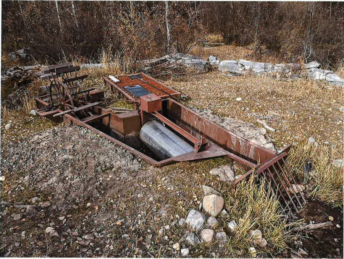
Photo 3: Fish screen structure
