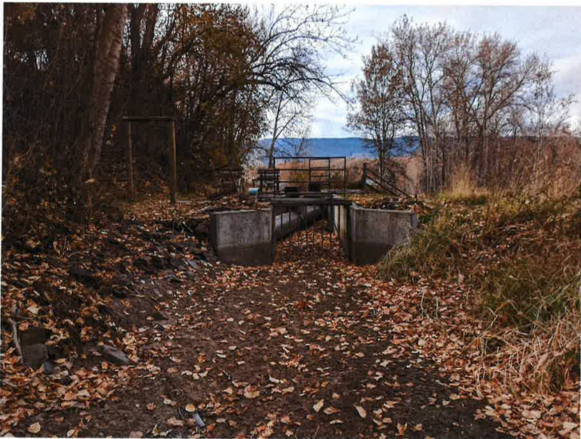
Photo 2: Fish screen/bypass approach
