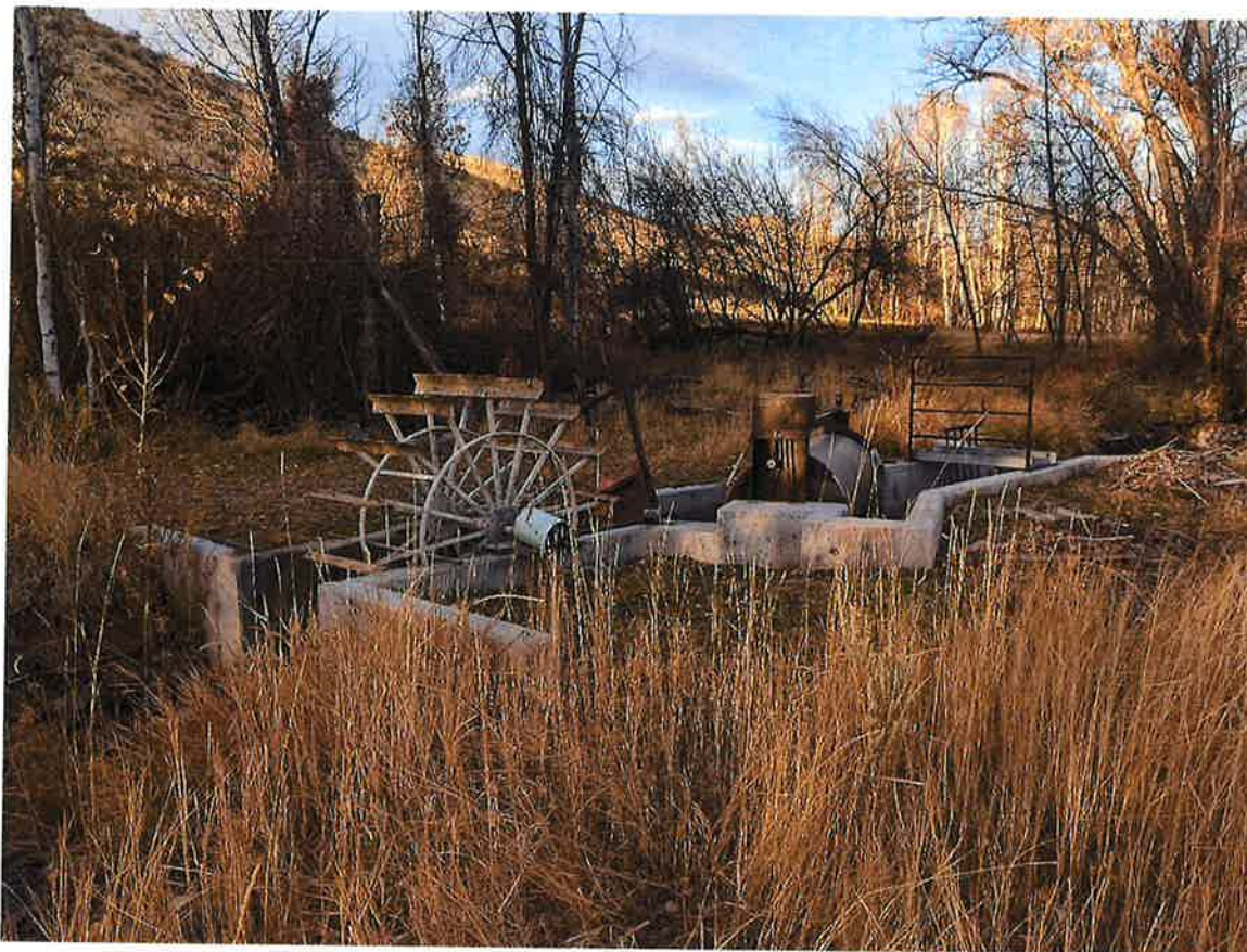
Photo 3: Fish screen structure
