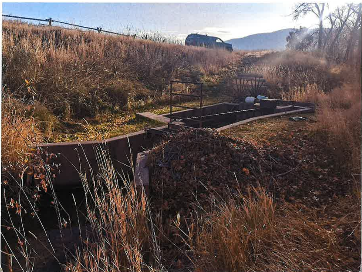
Photo 2: Fish screen/bypass structure
