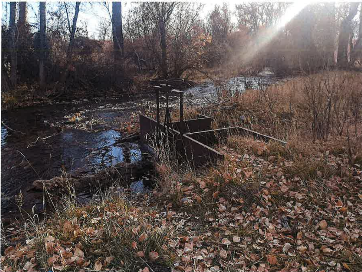
Photo 1: Diversion on Carmen Creek
