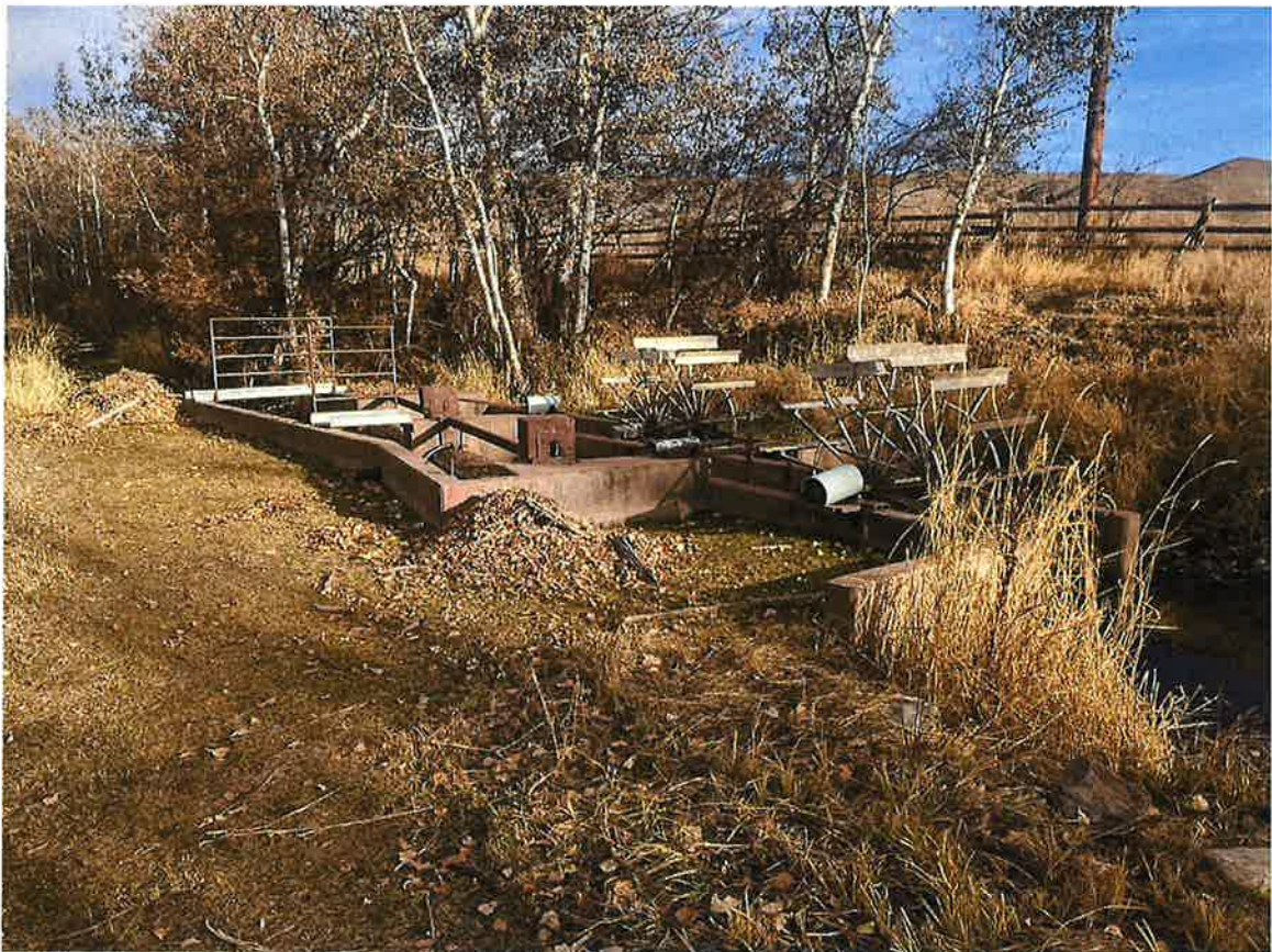
Photo 3: Fish screen structure
