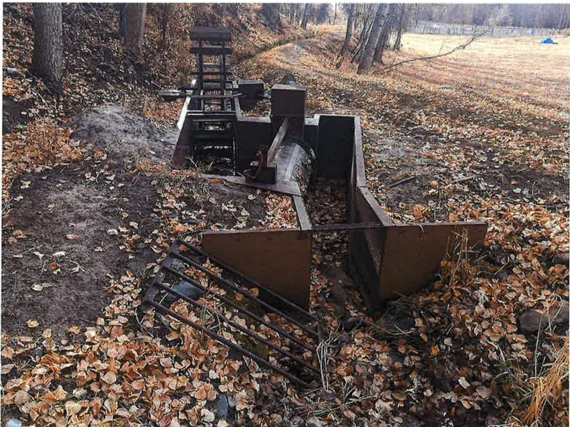
Photo 2: Fish screen/bypass structure
