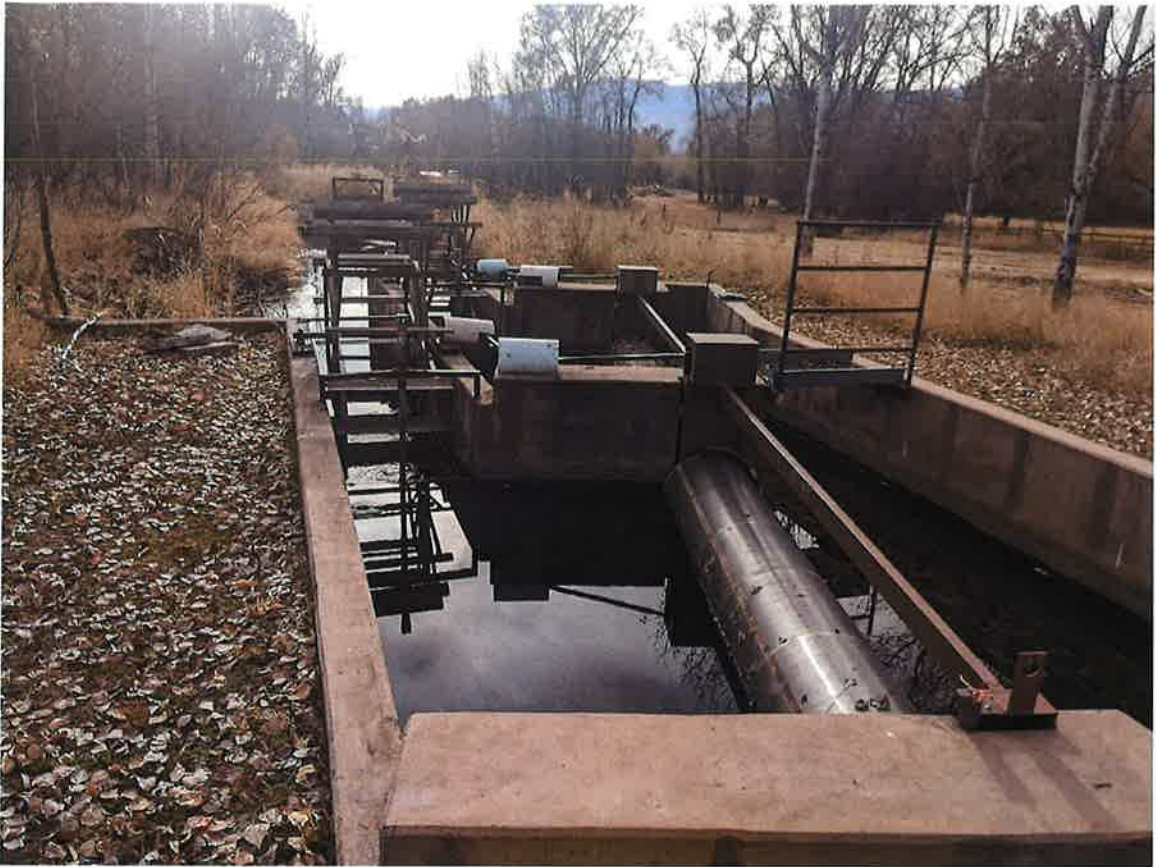
Photo 3: Fish screen structure
