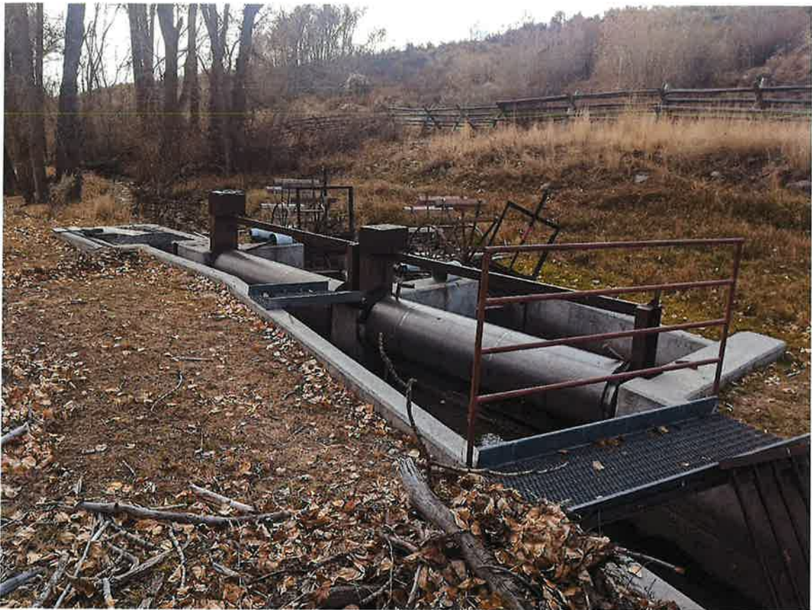
Photo 3: Fish screen structure
