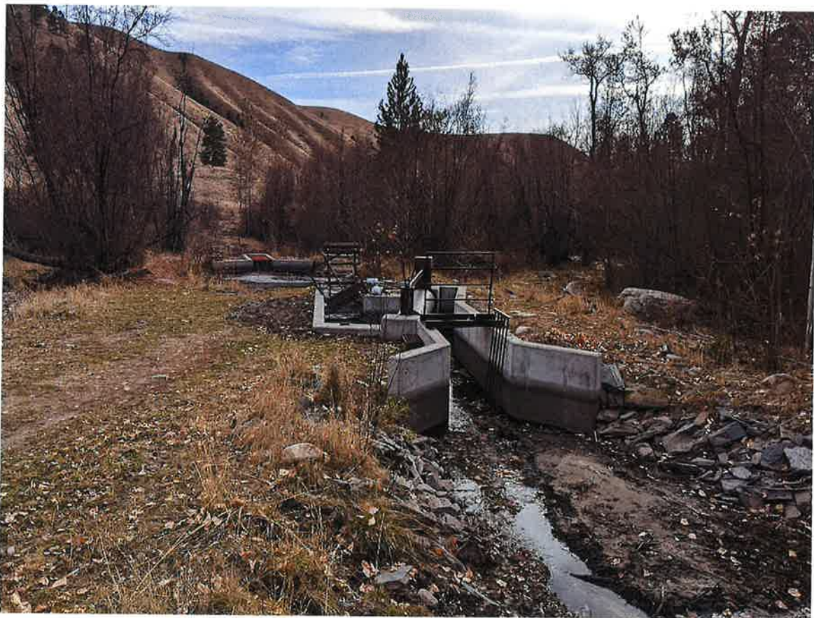
Photo 2: Fish screen/bypass approach
