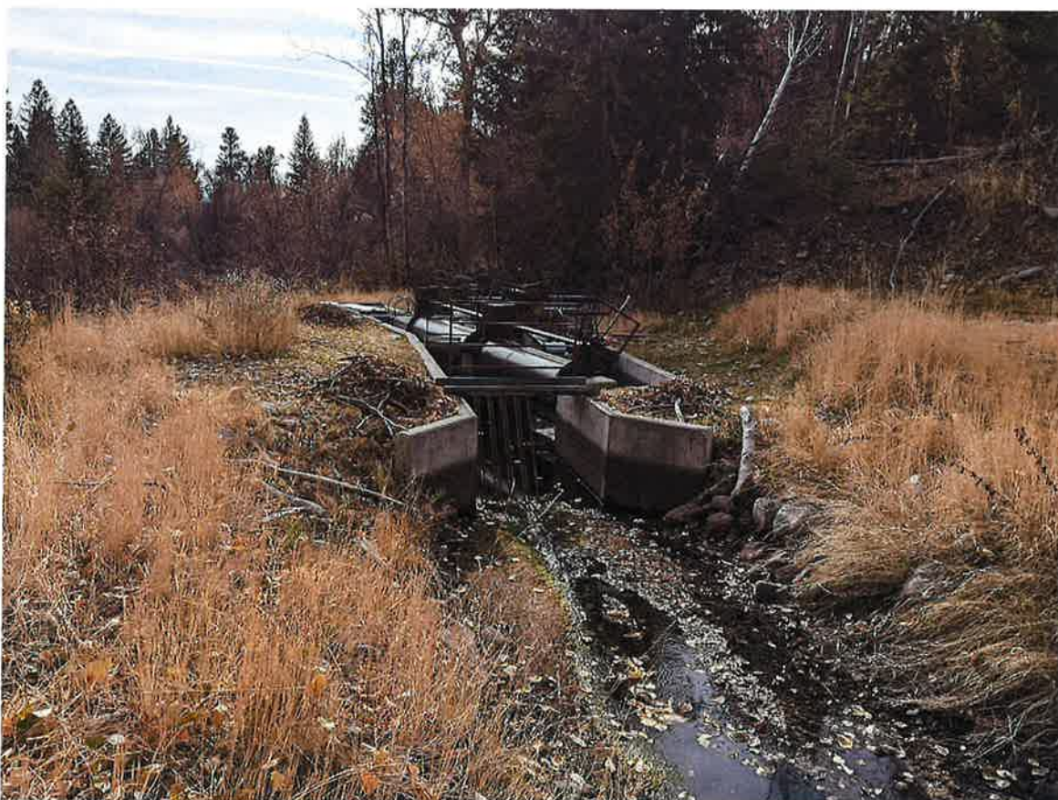
Photo 2: Fish screen/bypass approach
