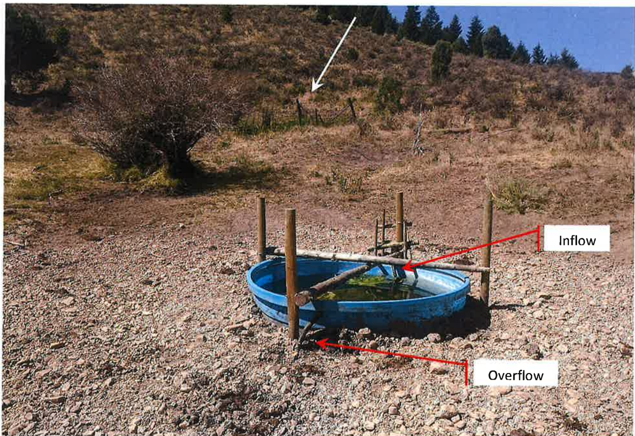
Photo 2: View of the trough filled by the spring shown in the previous photo, depicting the locations of the inflow and overflow pipes. The spring is visible in the background, indicated by the white arrow.
