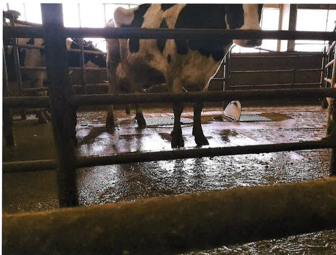
Looking at deck flush holes within the dairy's milking parlor.
