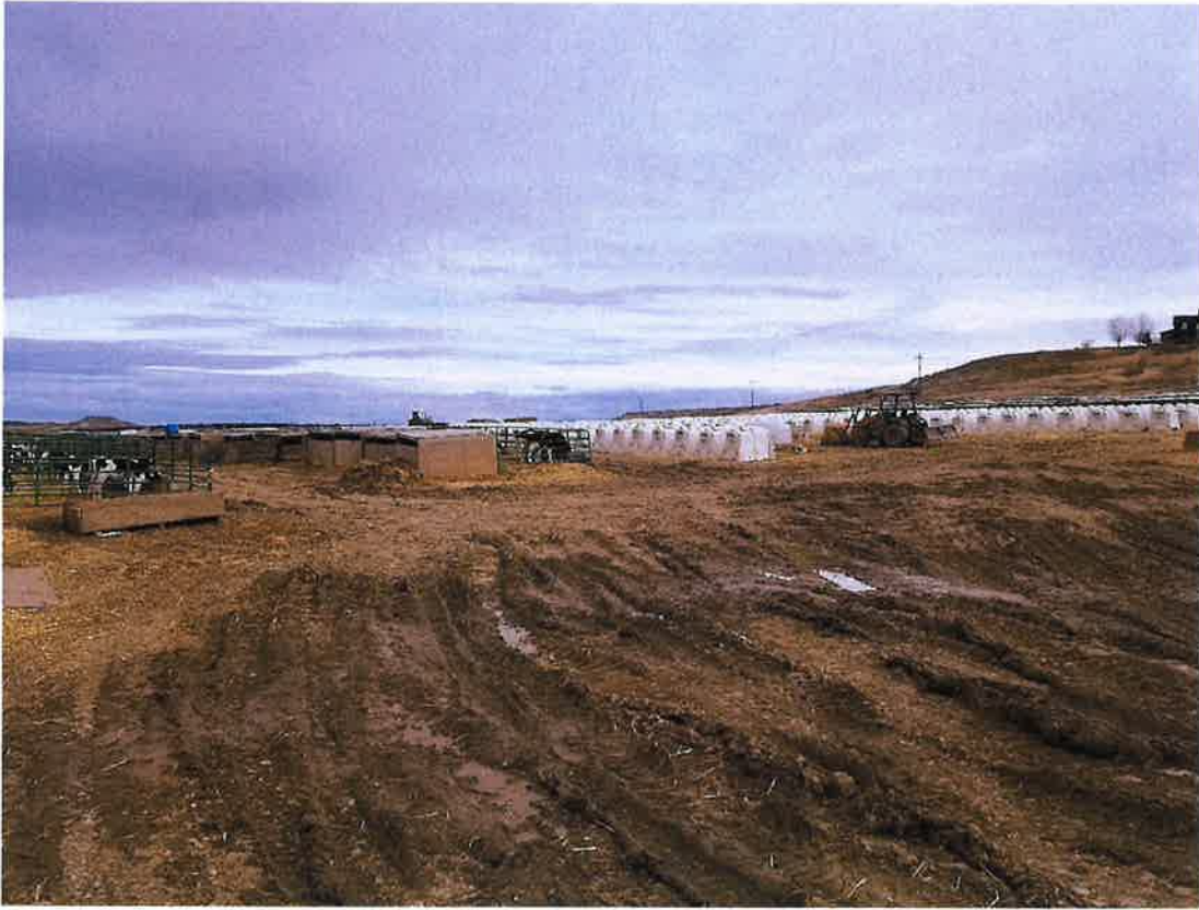
Looking at holding pens and beds for approximately 2,500 heifers located up the hill from main dairy.
