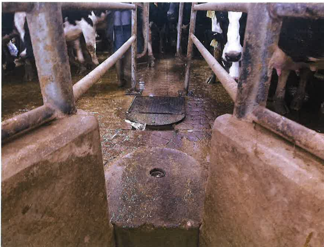
Looking at deck flush holes within the dairy's milking parlor.
