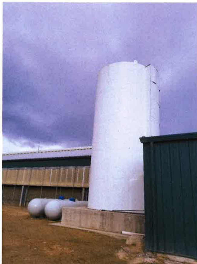
Looking at holding tank for well water and treated water from the Snake River used for dairy operations.
