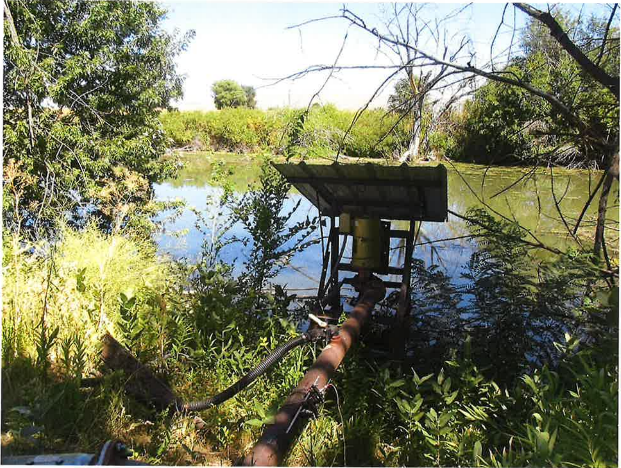
This 30 hp Baldor Pump diverts water from a slough of the Snake River located at the northeast edge of the farm. The Panametric measuring device can be seen on the pump.
