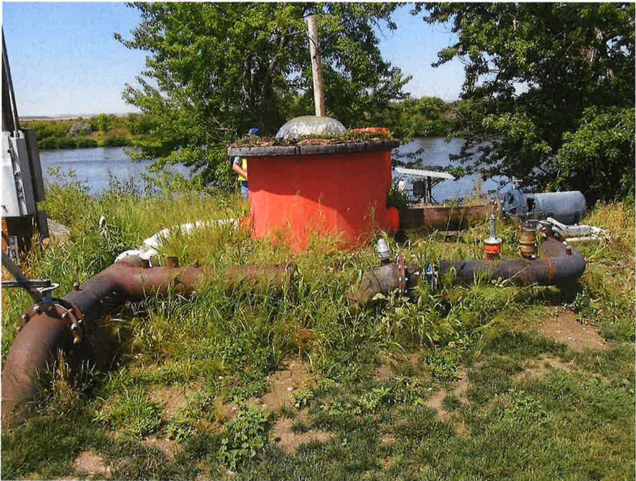
Photo of bubbler. The pipe to the left leads to the gated pipe which irrigates the 20 acres south of the farmhouse. The 25 hp booster pump (also see photo below) on the left pressurized the three pivots irrigating the field north of the farmhouse.
