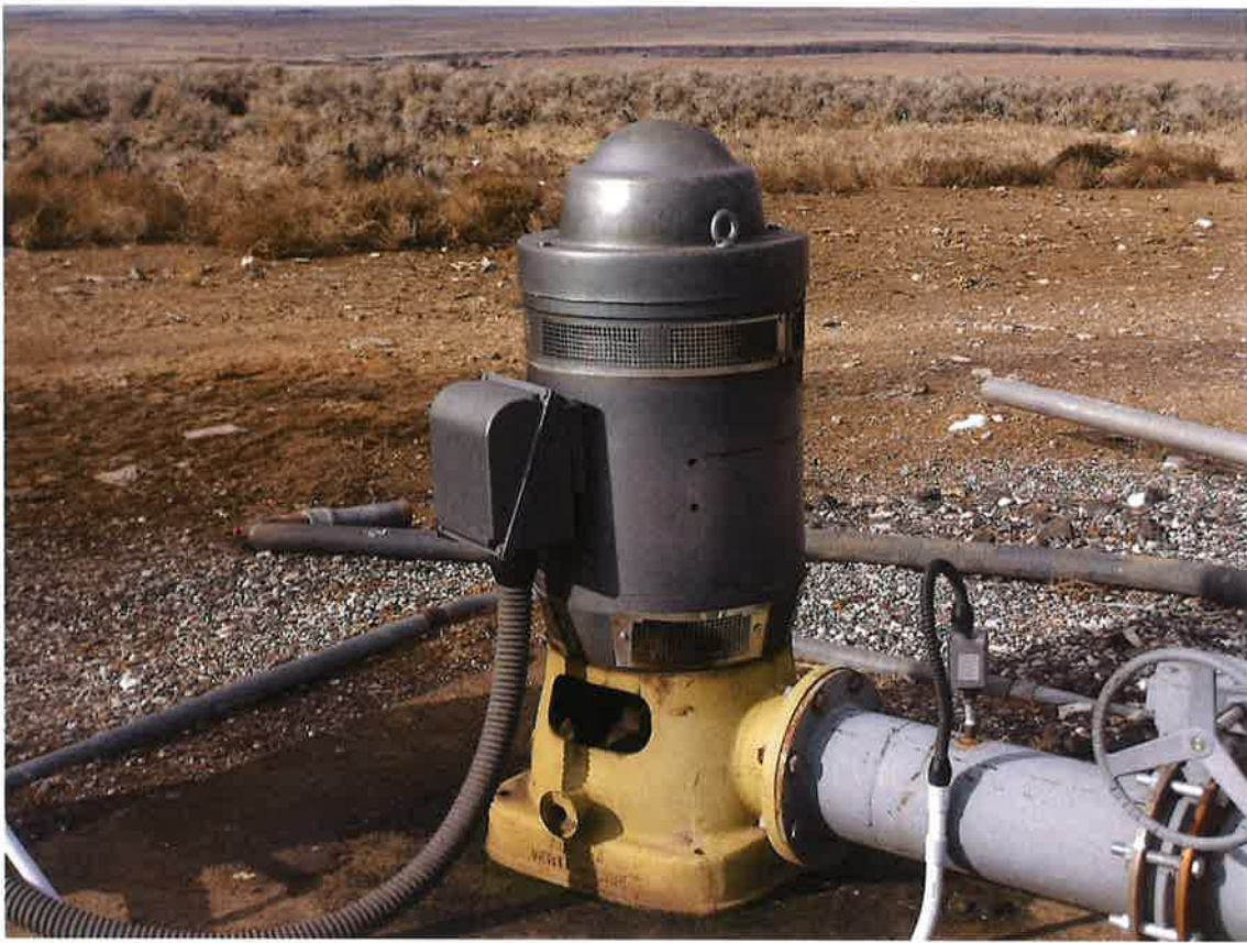
Point of Diversion
