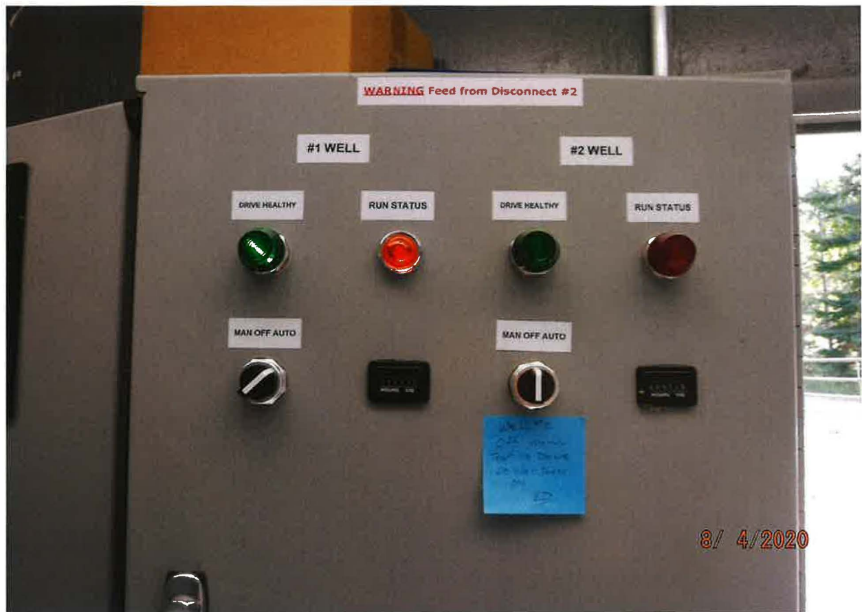
WELL PUMP(S) CONTROL PANEL & ELECTIC WORKS
