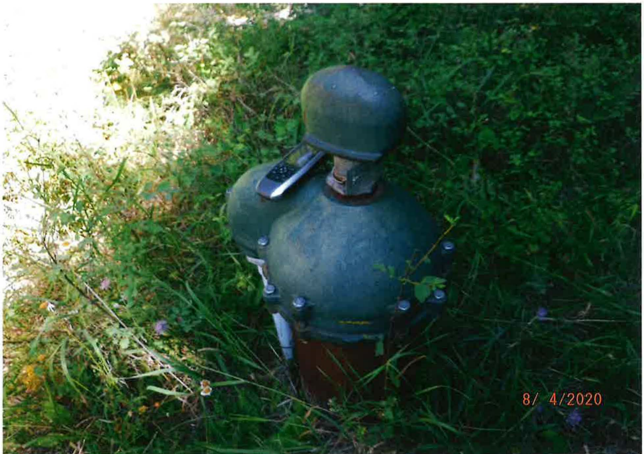
POD WELL No. 2 – NO TAG, 7.5 HP PUMP
