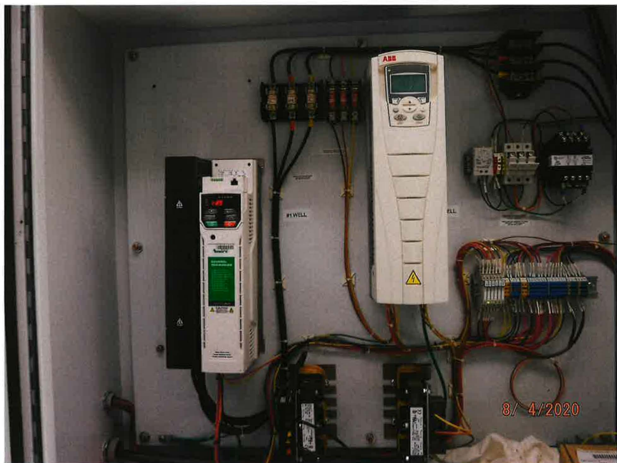
WELL PUMP(S) CONTROL PANEL & ELECTIC WORKS
