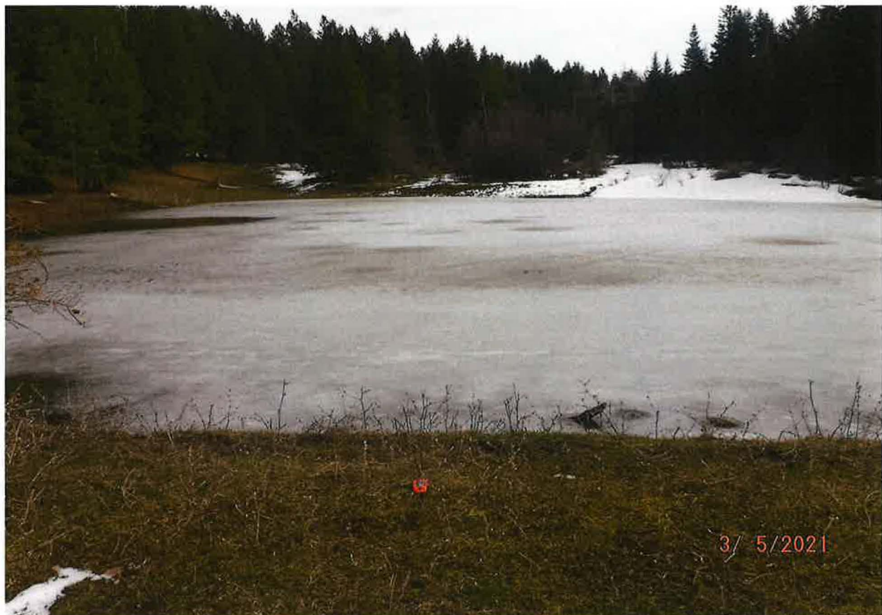
POD – EARTHEN DAM CAPTURES UNNAMED STREAM WATER IN POND
