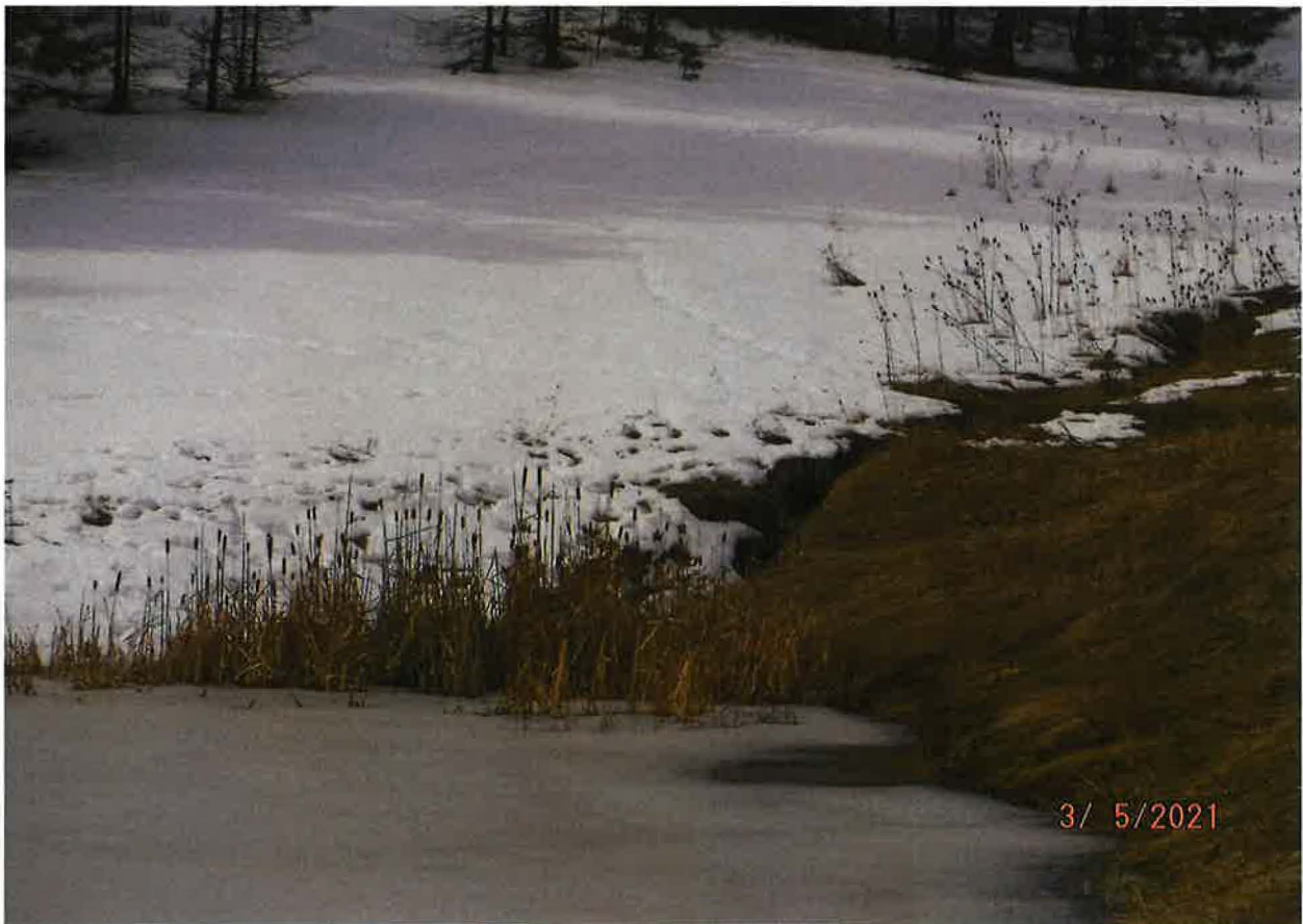
SURFACE RUNOFF WATER INFLOW TO POND
