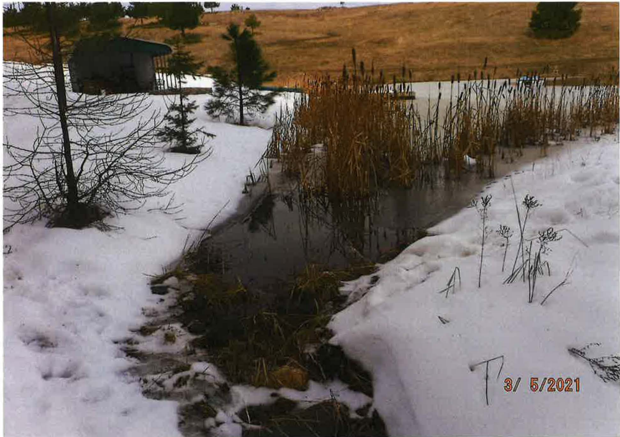
SECONDARY OVERFLOW FROM POND – ROCKED IN CHANNEL
