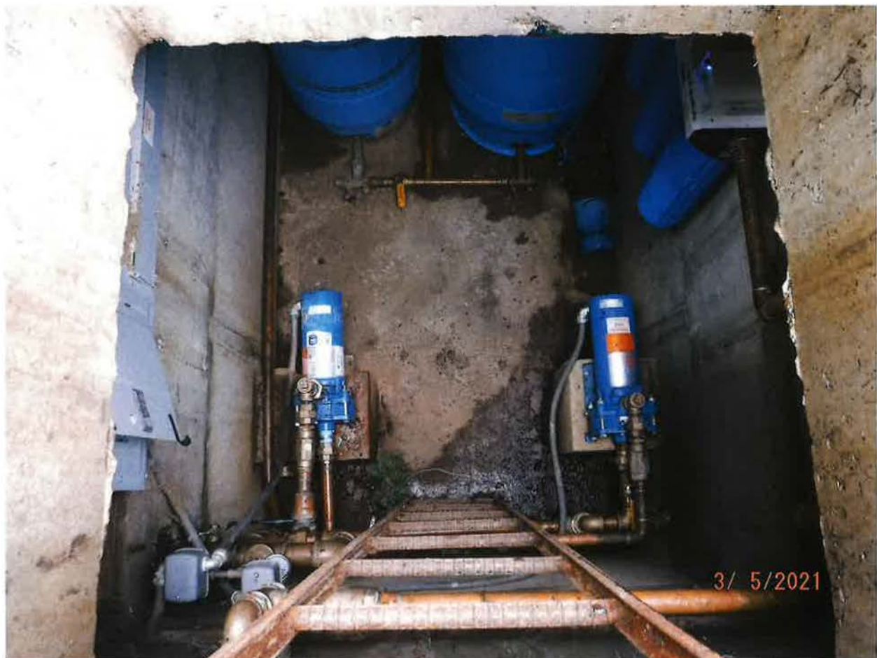
VAULT FOR 2EA DISTRIBUTION PUMPS, FILTRATION, AND PRESSURE TANKS FROM STORAGE RESERVOIR
