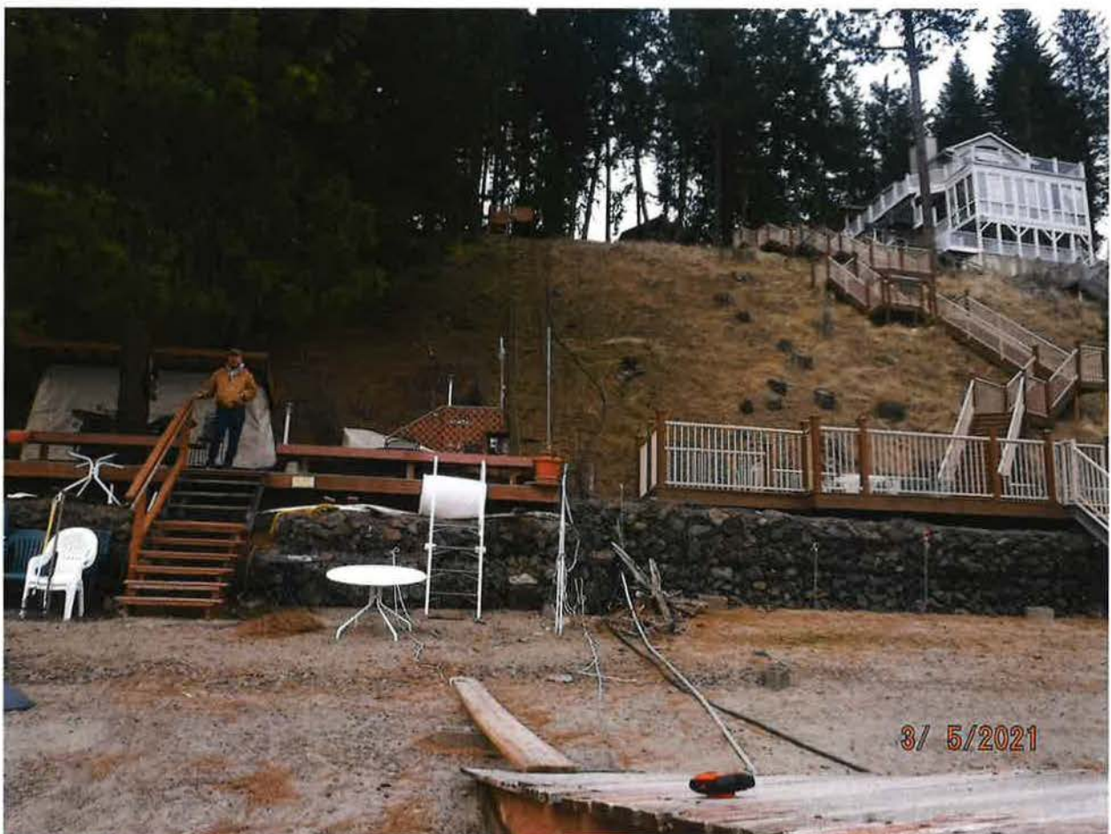
LOW WATER ~ PIPE ROUTES ALONG DOCK UP SHORE AND UP HILL TO STORAGE TANK
