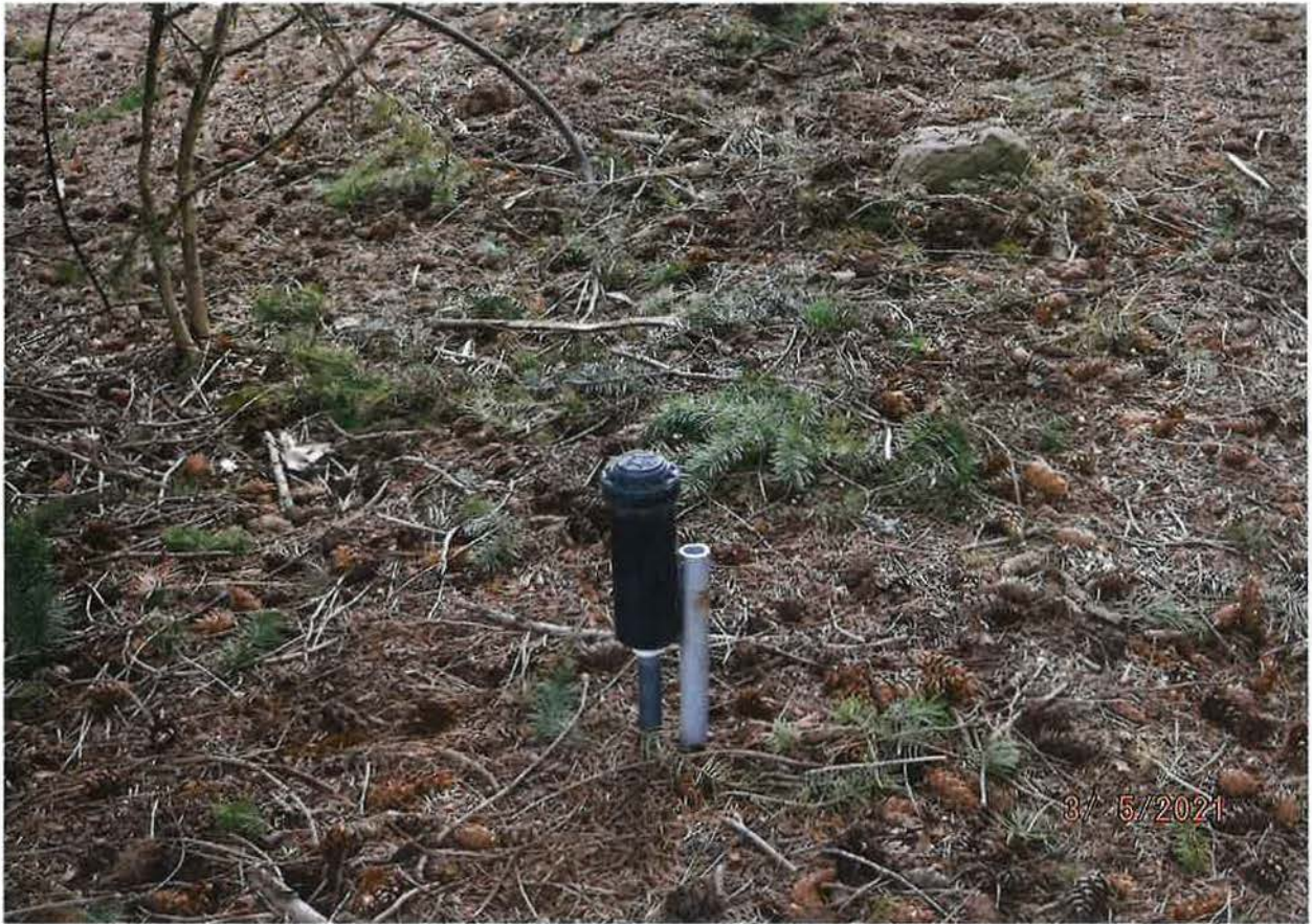
IRRIGATION UP TO ½ ACRE BY HOSE AND SPRINKLER & PRESSURIZED IRRIGATION SYSTEM
