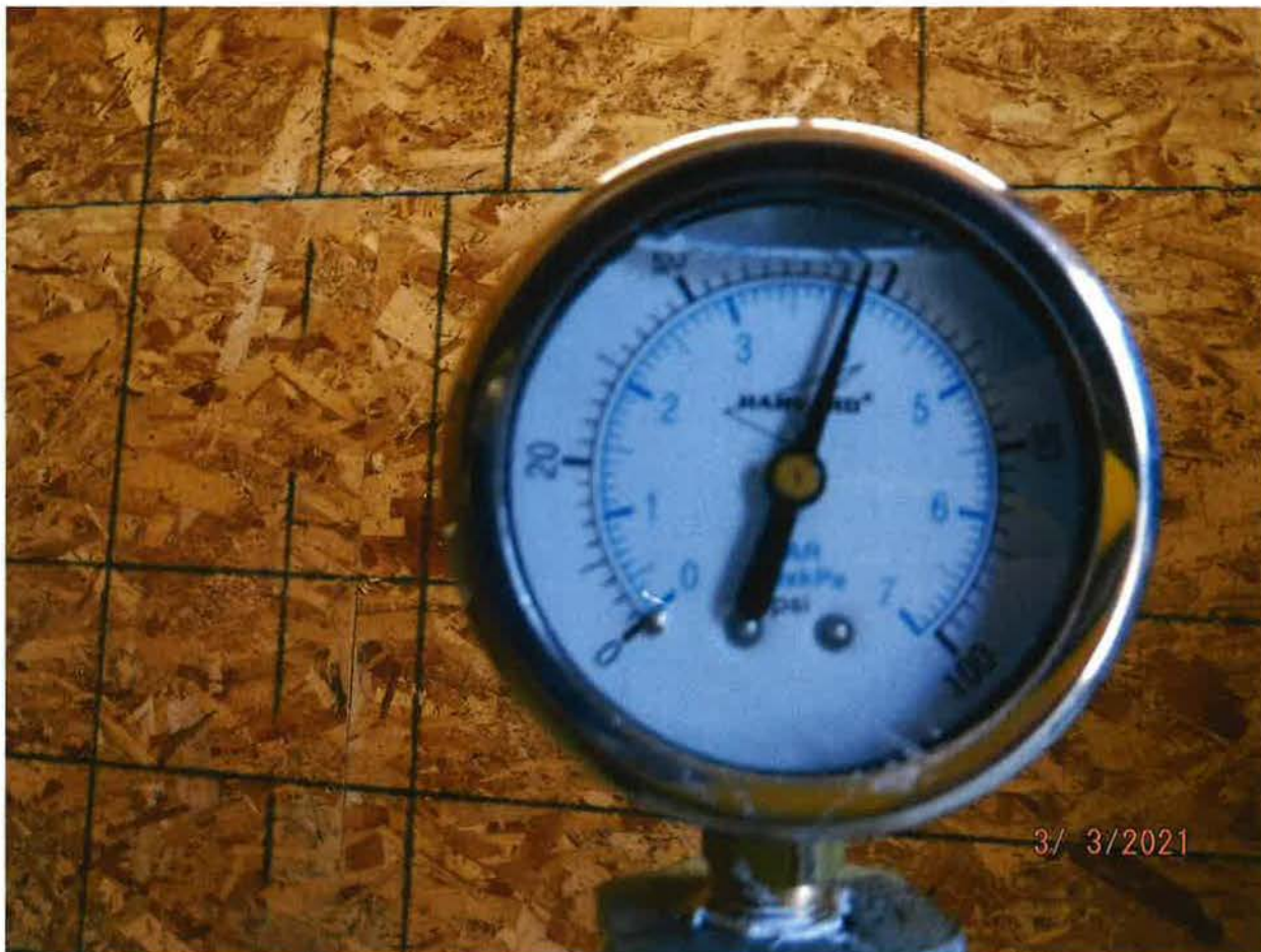
WATER SYSTEM OPERATES AT 55 PSI
