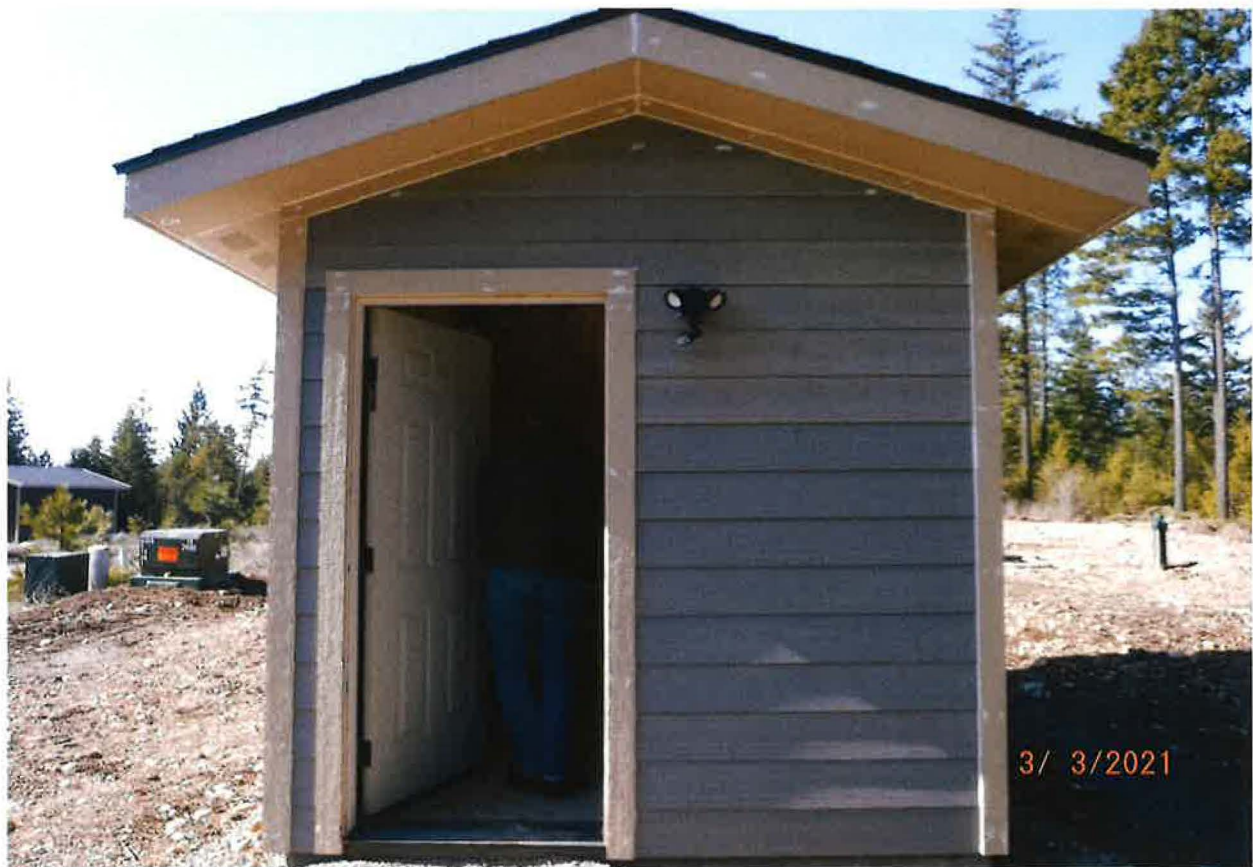
PUMP STATION CO-LOCATED WITH WELL
