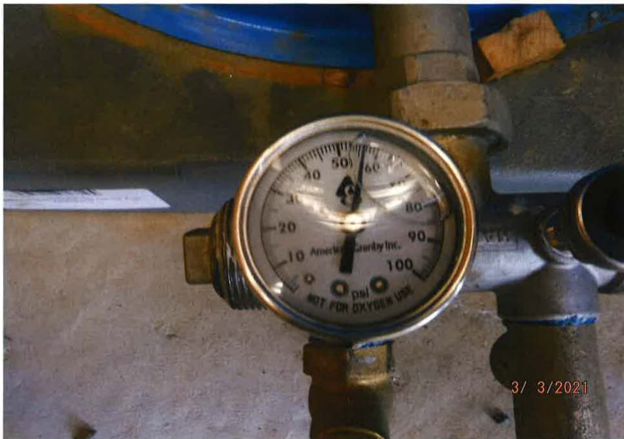
WATER SYSTEM OPERATES AT 55 PSI
