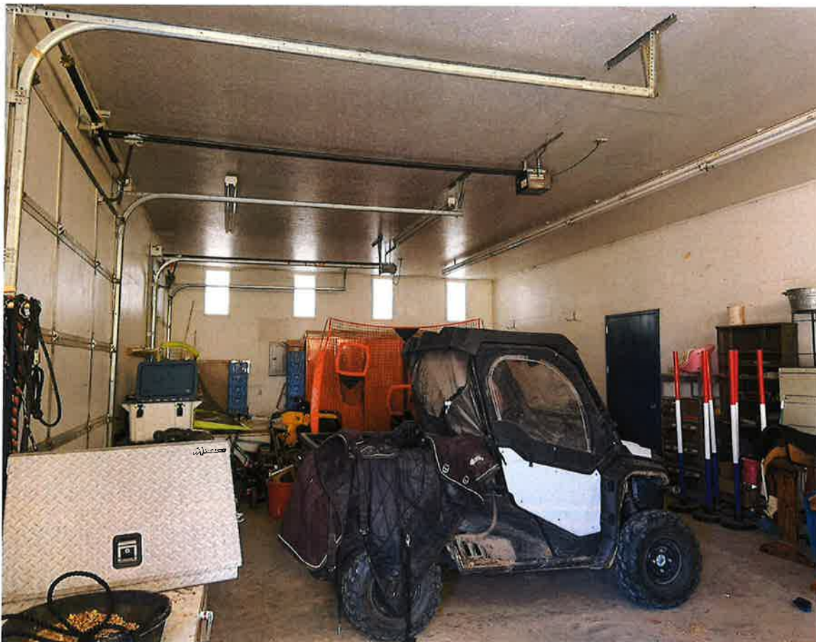
Fig. 2 – Inside of shed where heating/domestic is used. Barn, also heated, is accessed through blue door on right side of picture.
