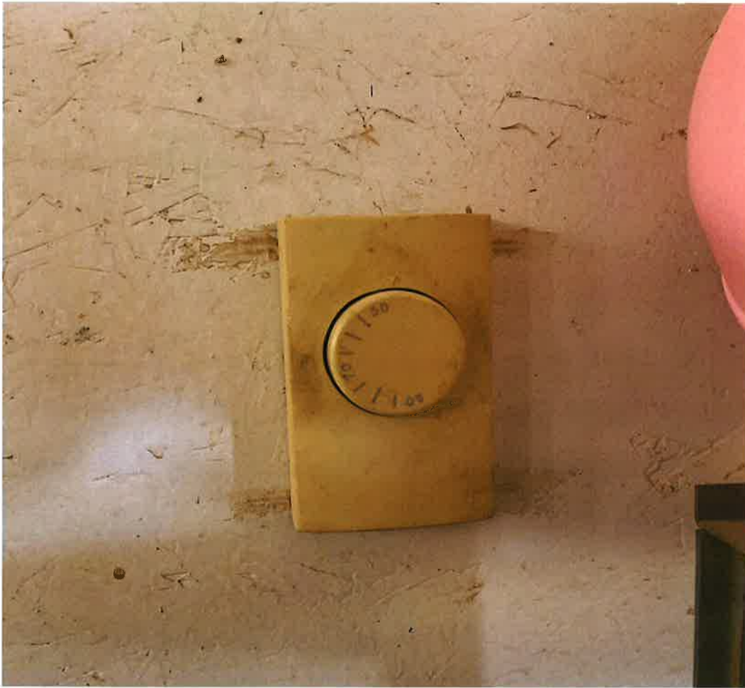
Fig. 3 – Thermostat in the shed/barn using geothermal heat is kept between 50° - 65° F during colder months.
