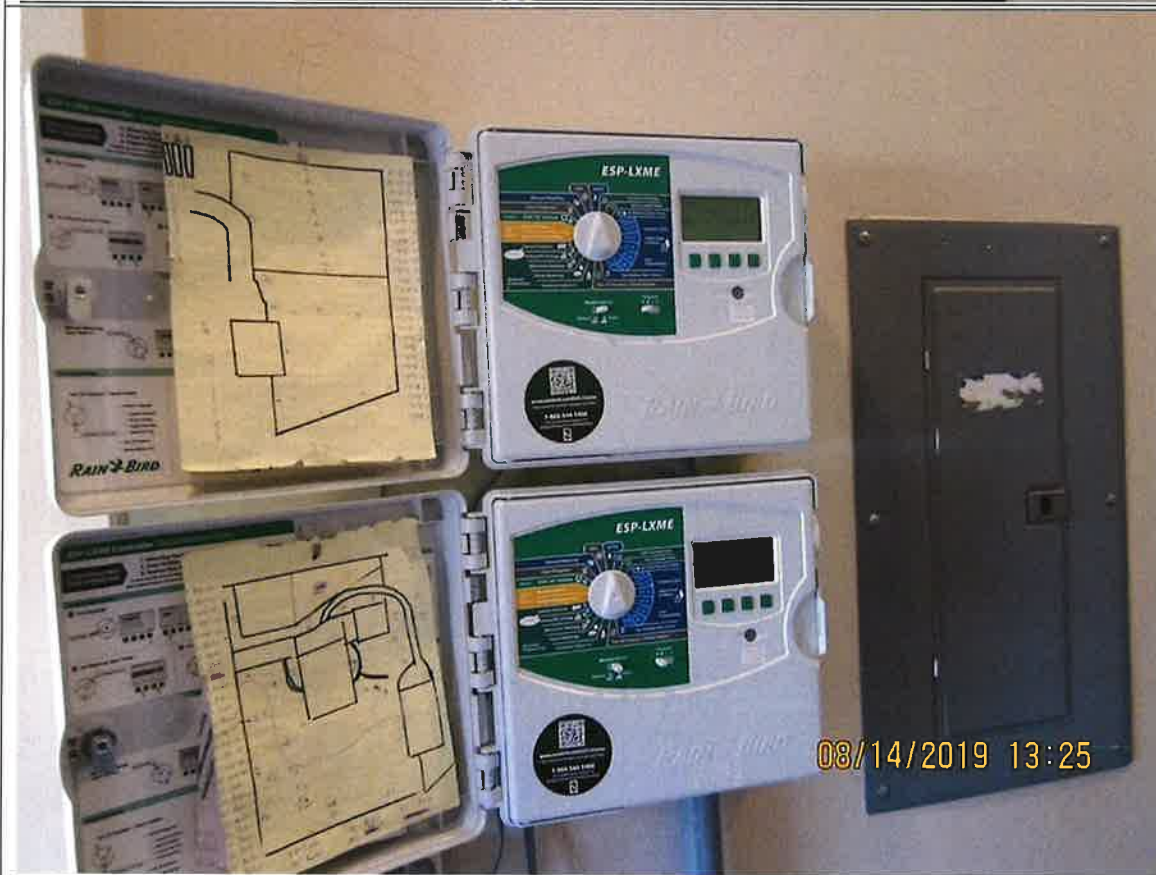
Figure 4. The dual Rainbird programmable zone controllers manage 33 zones for the lawn/residential area and 23 zones for the pastures.
