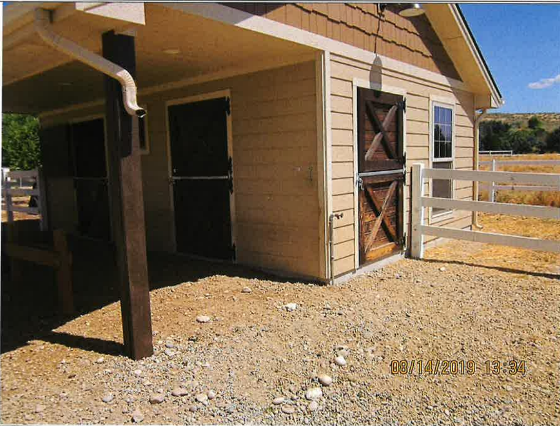
Figure 8. Stockwater development is composed of spigots near barns and corrals.
