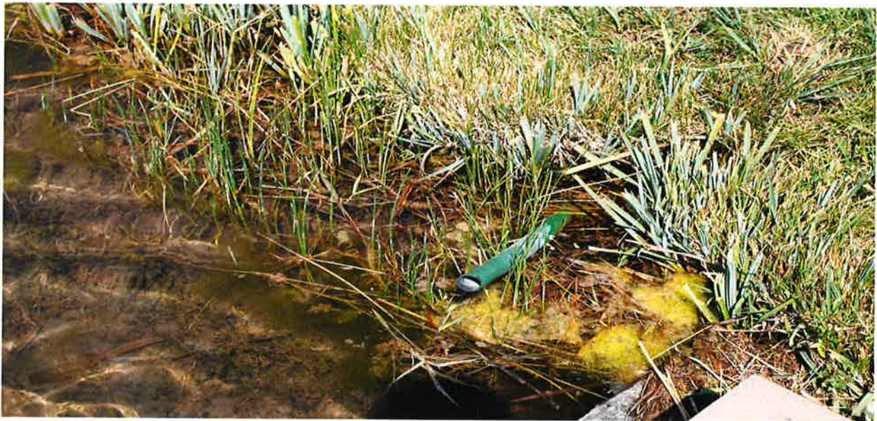
Pipe in pond #2
