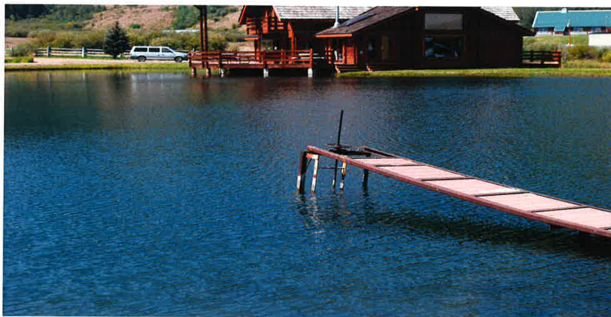
Headgate and culvert in Pond #2
