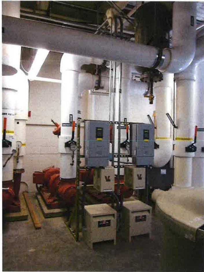
Figure 3: Additional drives in the distribution system
