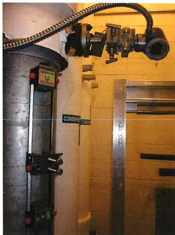
Figure 6: Veris Veribar Flow Meter
