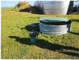
Well head next to vertical culvert.
