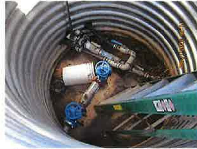
Diversion works in vertical culvert.
