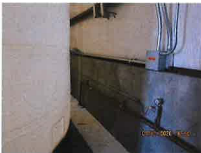
1" line with pressure gage.
