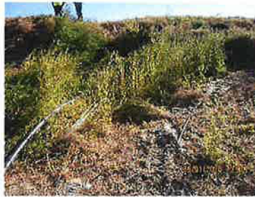
4" pipe from well as it exits hillside and leads to the pond.
