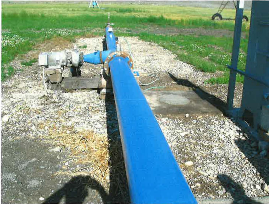
Photo 3. Looking westerly along mainline. Booster pump on left was not used during field exam measurement. Old well plug visible right center of photo.
