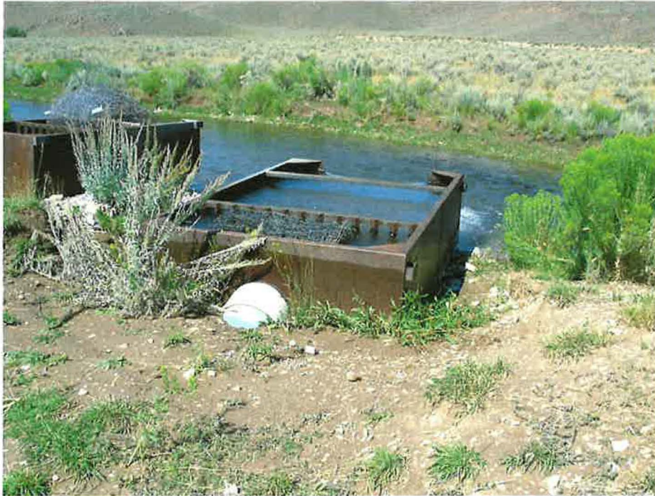
Photo 5. Discharge end of mainline with weir used to measure pumped discharge. Wire and vertical bars used to dissipate energy & calm flows to improve measurement.
