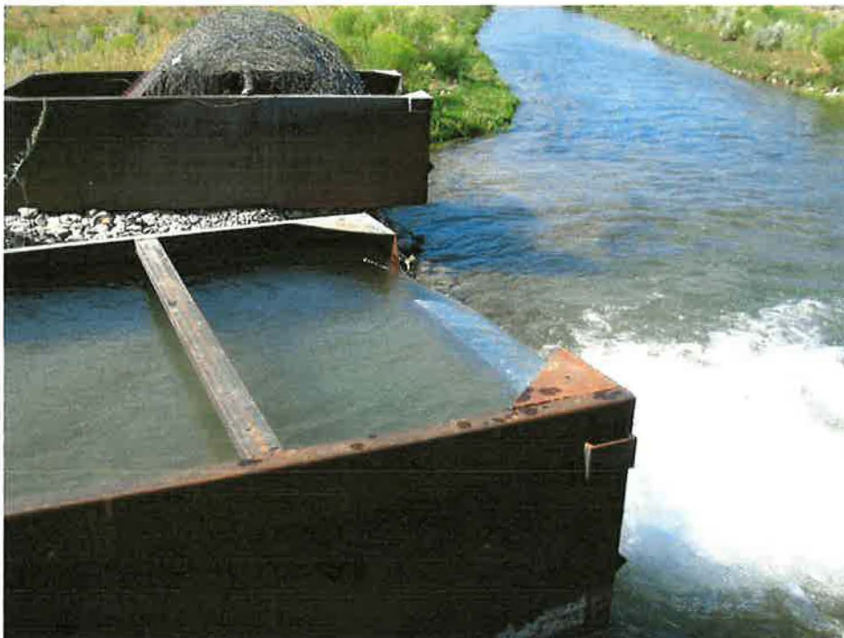
Photo 6. Weir discharge and weir pool showing reasonably uniform flow approaching the weir crest.
