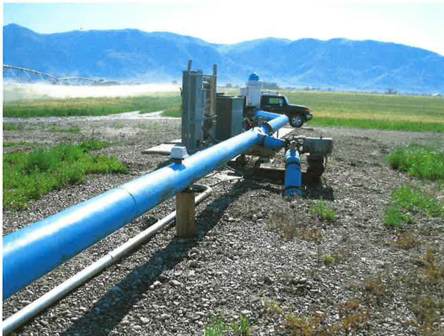
Photo 2. Looking back toward well and pump along mainline. Meter in mainline is not used.
