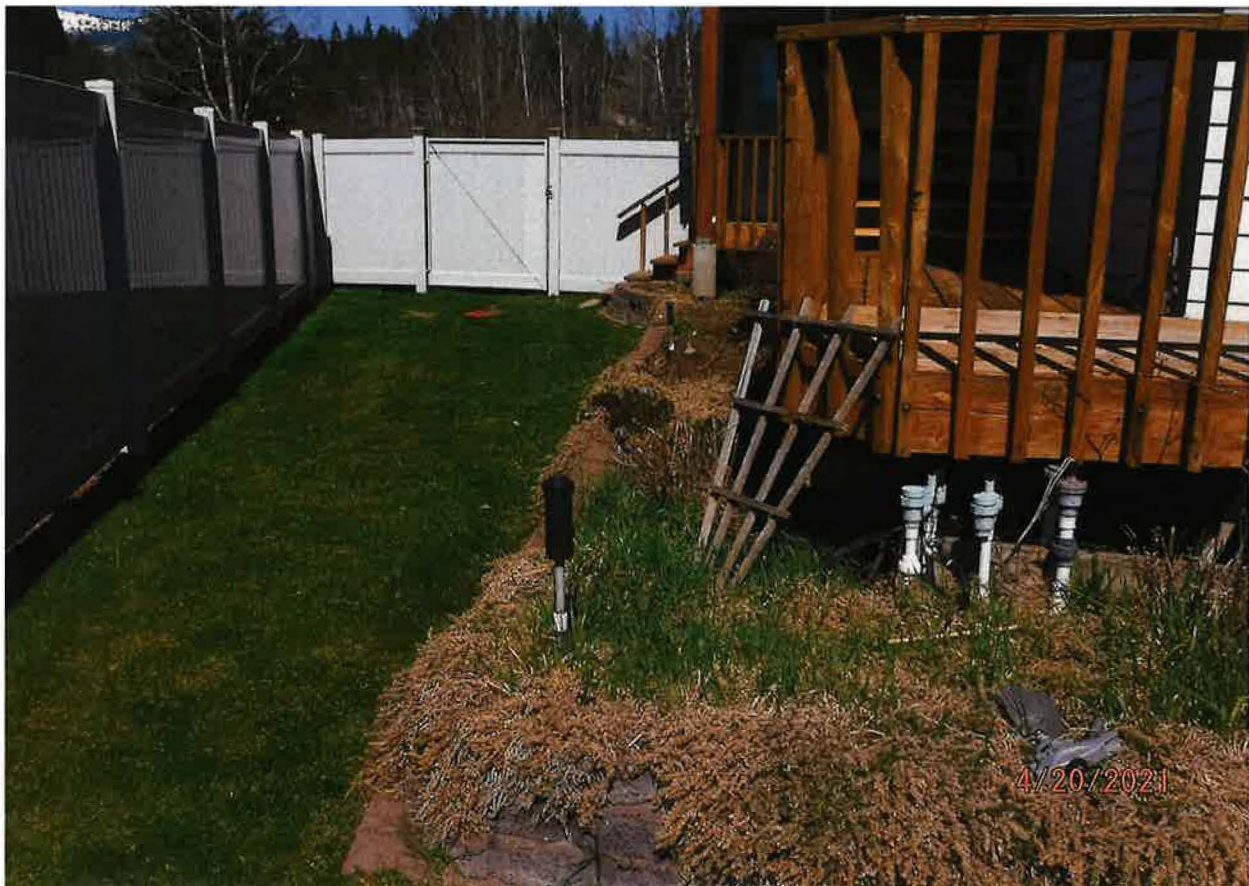
IRRIGATION POU – PRESSURIZED SPRINKLERS
