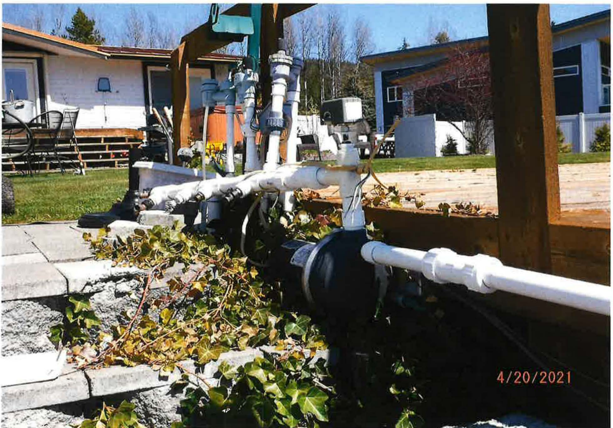
WATER SYSTEM WORKS – MULTIPLE ZONE STUBS AND 1.5 HP PUMP
