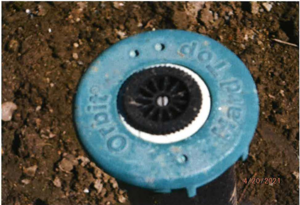
PRESSURIZED SPRINKLERS USED AT POU
