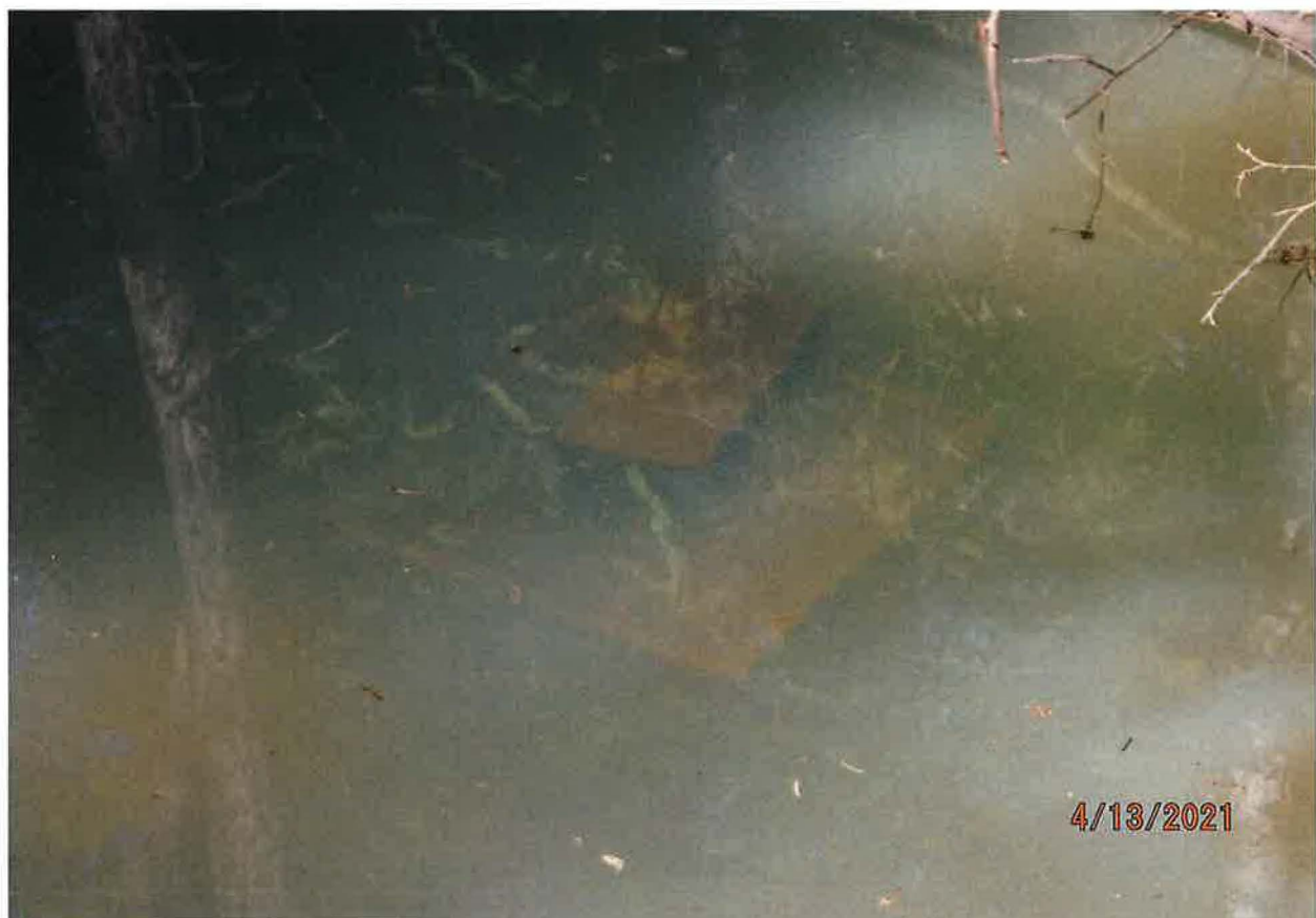
POD – SPRING BOX WITH 2 INCH POLY PIPE DIVERTING WATER FROM A 24-HR IMPOUNDMENT BASIN
